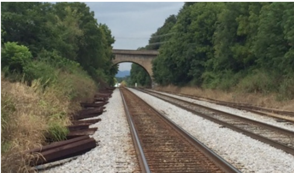
Figure 7: View looking west from the locally preferred site on the south side of the tracks. The mainline is the left most track.
