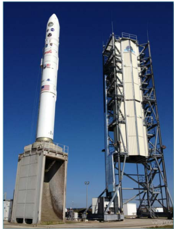
Figure 2-2. Pad 0B Small Class Solid Facility. Pad 0B is a state of the art launch pad for small solid fueled launch vehicles. The LADEE mission to the moon is shown.
