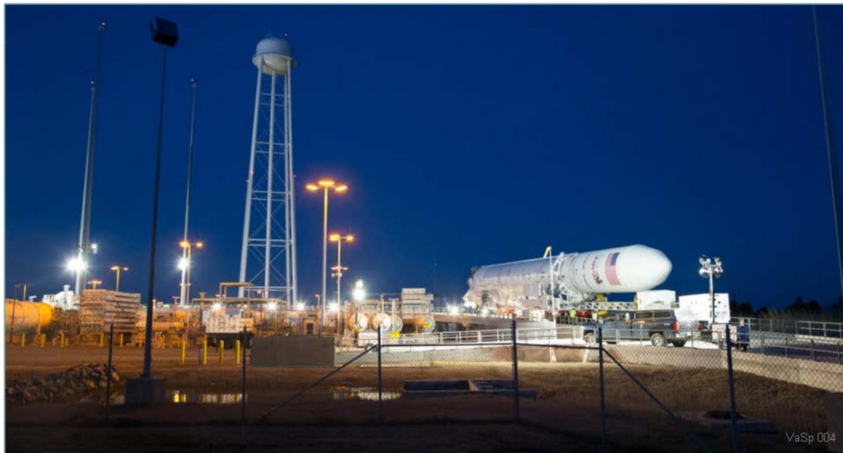
Figure 2-1. Pad 0A Medium Class Liquid Facility. Pad 0A is a state of the art launch pad for medium class liquid oxygen/kerosene launch vehicles.
