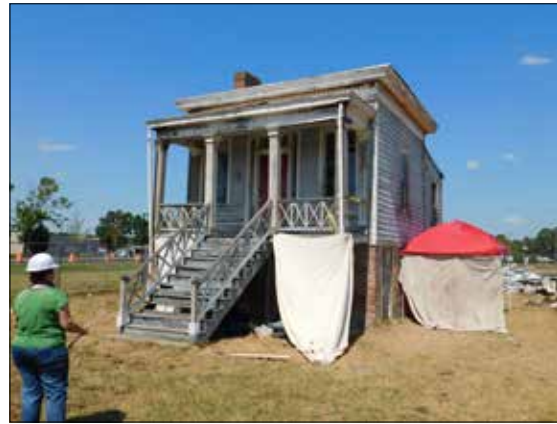
Restoration also included re-pointing the brickwork of the basement and foundation.
