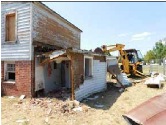
A backhoe removes a modern rear addition on the historic dwelling.
