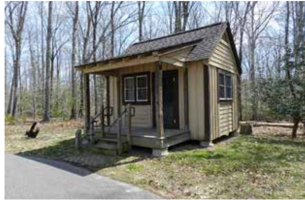
A contributing building in the Pocahontas State Park Historic District.
