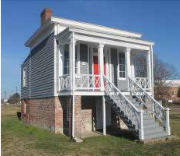
Summerseat after the first phase of restoration by HistoriCorps volunteers, completed in October 2016. (Photo: HistoriCorps)
