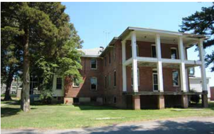
Piedmont Geriatric Hospital, completed 1918.
