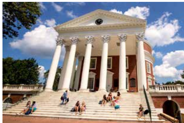
After two years undergoing extensive renovations, the Rotunda at UVA re-opened in September, 2016. (Photo: UVA)
