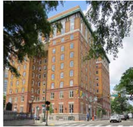
The former Ninth Street Office Building was renovated and renamed the Barbara Johns Building in early 2017. (Photo: DGS)
