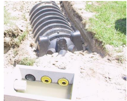
Gravelless Material Installation
