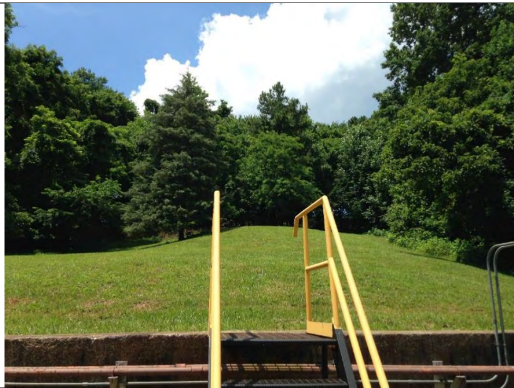
Photo 3-6 Location of former 100,000-gallon No. 6 Heating Oil AST at the boiler plant, Building 77. AST removed in 1999.
