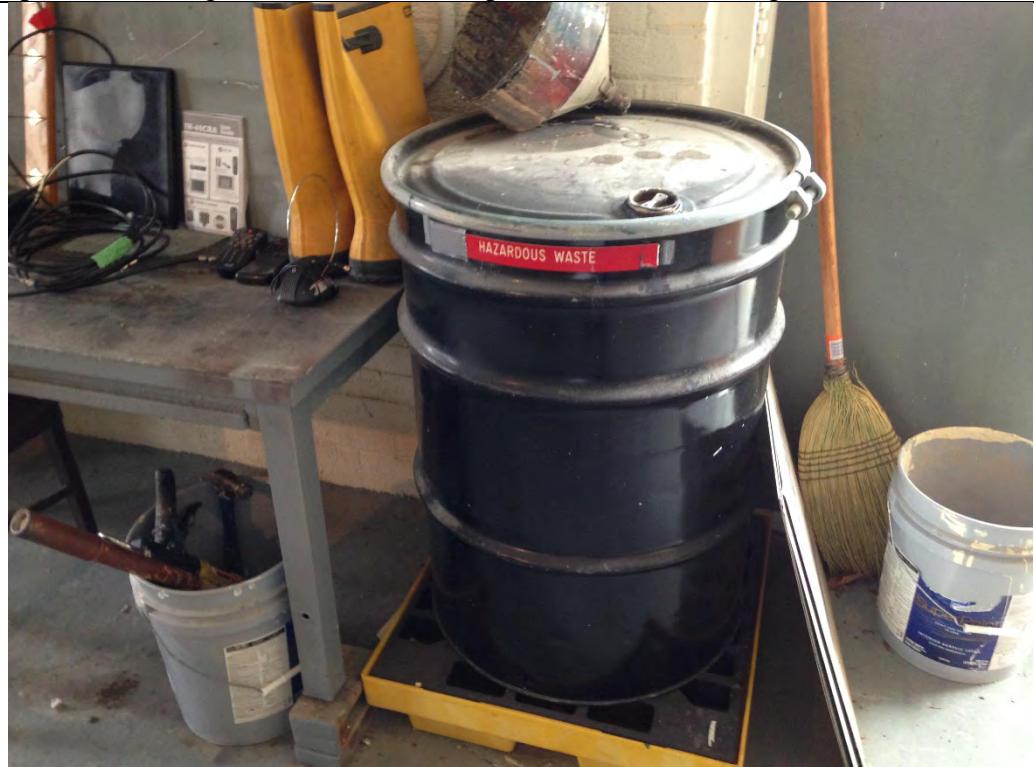
Photo 8-3 Spent paint thinner and solvent storage as hazardous waste within Building 82. No evidence of spills or staining, and no floor drains present within building. Minimal accumulation, and when full the drum is properly disposed by an third party (Environmental Options).
