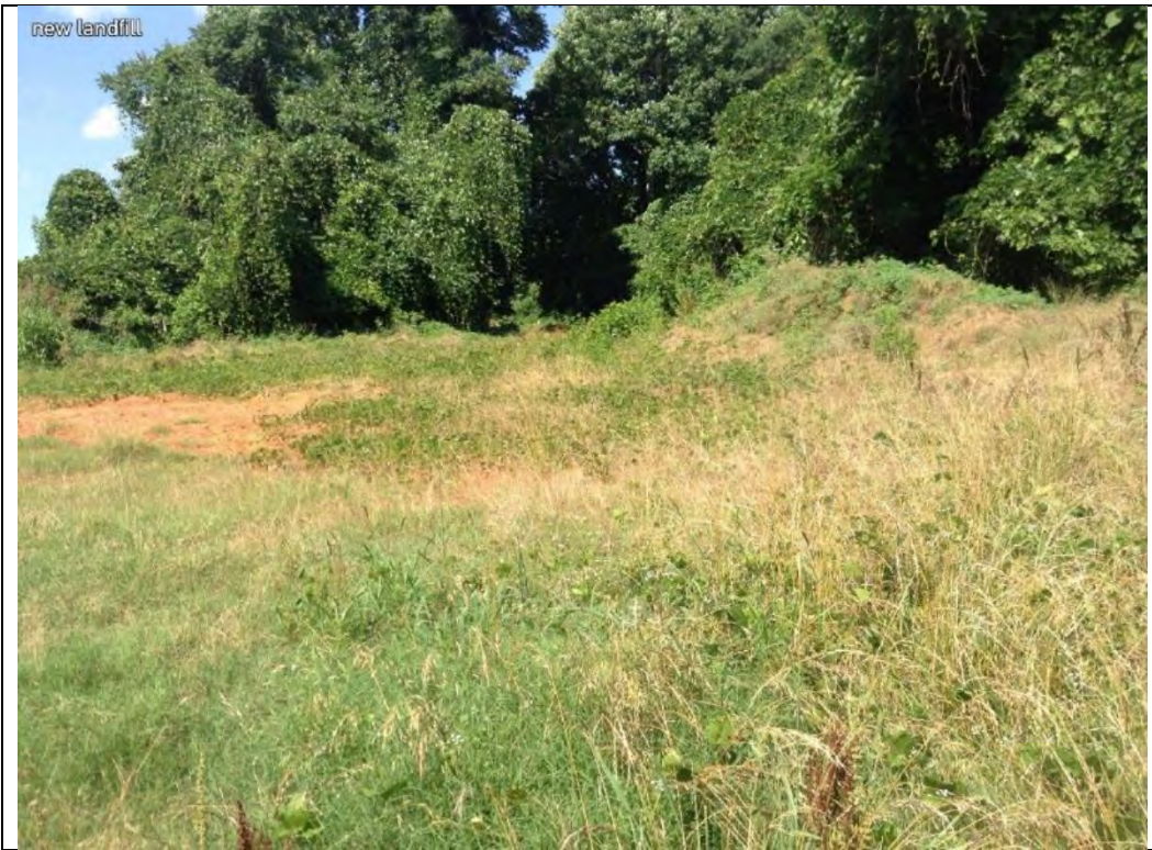
Photo 14-2 Fill area, former landfill, immediately south of the “ball field” scrap storage yard.
