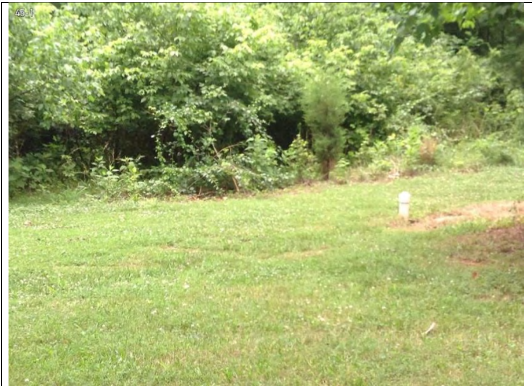
Photo 25-1 Septic cleanout and location of system behind Building 45. Typical example of similar systems observed throughout facility at Buildings 34-A, 48, and 66. Would need proper closure prior to demolition, but not an REC.
