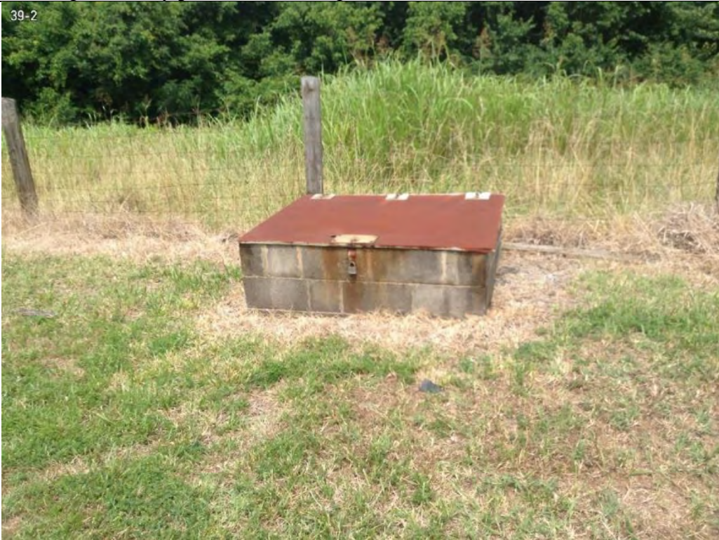
Photo 27-3 View of concrete block structure
