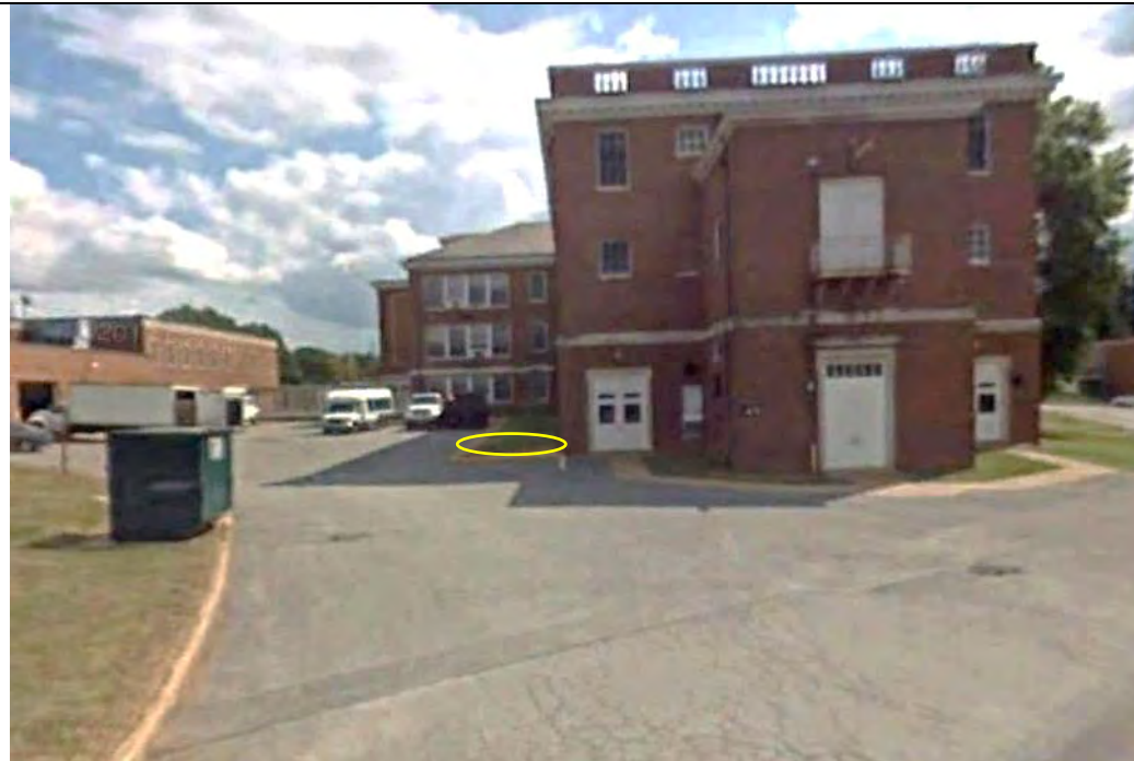
Photo 35-1 View of Building 49, former 1,000-gallon gasoline UST location as indicated by yellow oval
