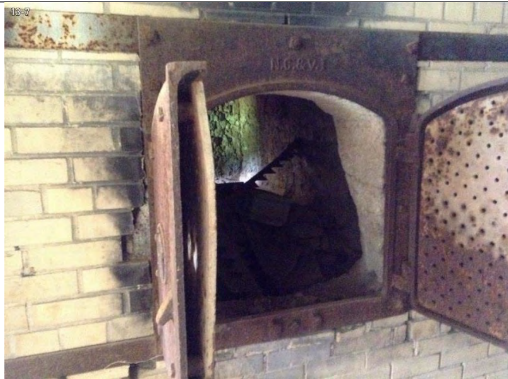
Photo 11-3 View into former incinerator, ground level.
