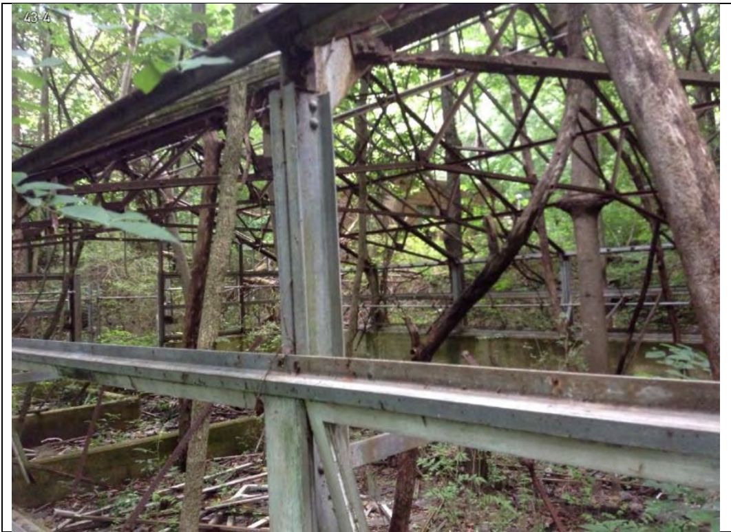
Photo 26-2 Close-up of sparging and treatment cells within old sewage plant
