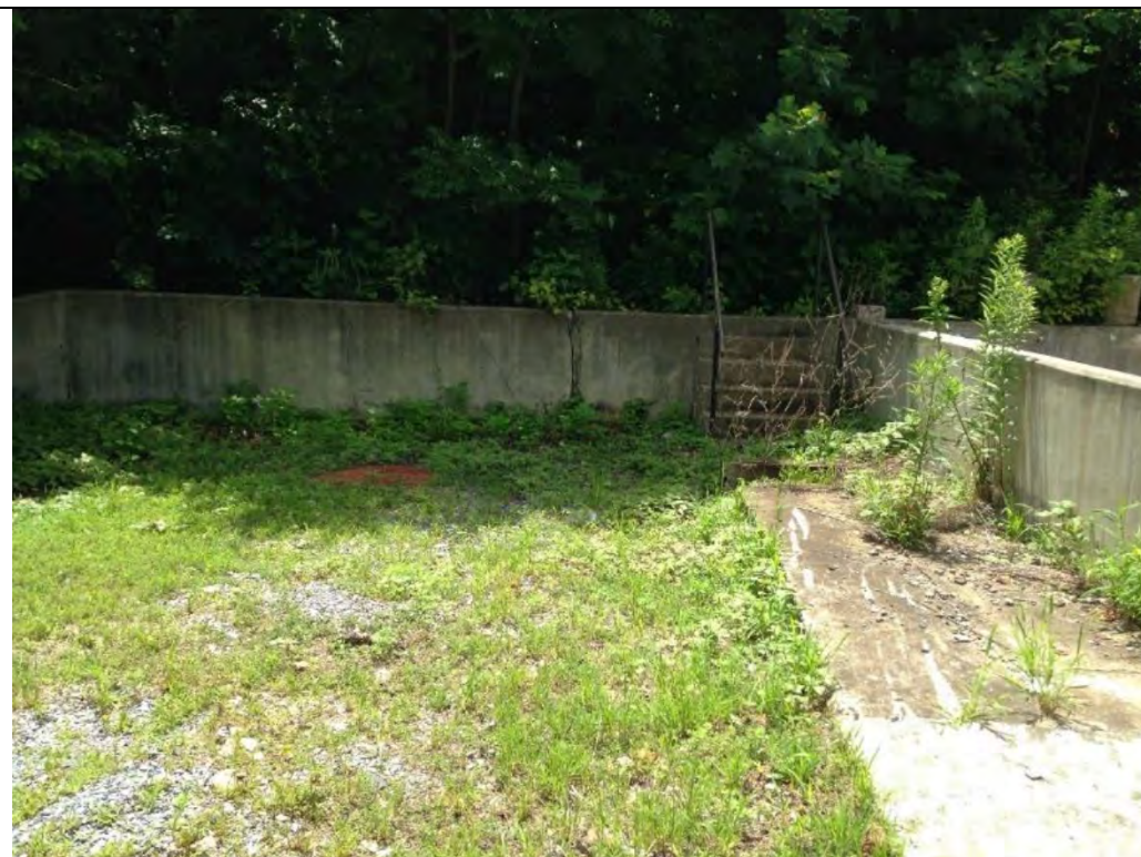
Photo 9-1 Apparent former coal bin at boiler plant (Building 77), no visual evidence of remaining coal or fines.
