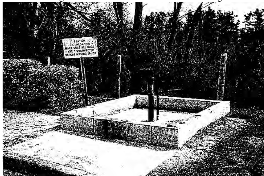
Photo 3-8 Location of former remote fill for 100,000-gallon No.6 heating oil AST as presented in the August 1999 AST Closure Report.
