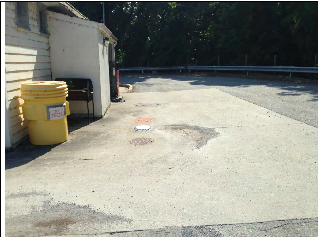
Photo 30-1 Location of 8,000-gallon gasoline UST at Building 36
