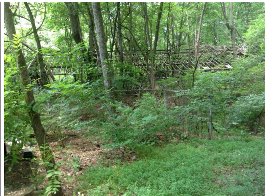
Photo 26-1 View of old sewage treatment plant Building 43
