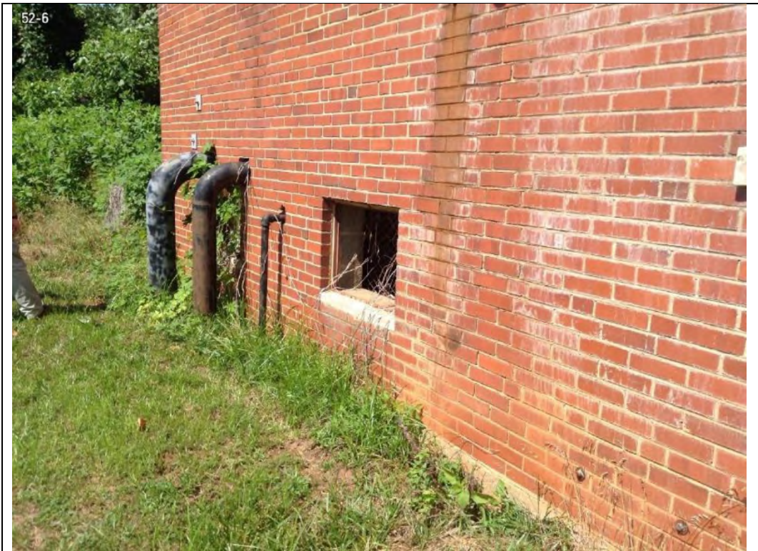
Photo 28-1 Unidentified underground utilities entering Building 53
