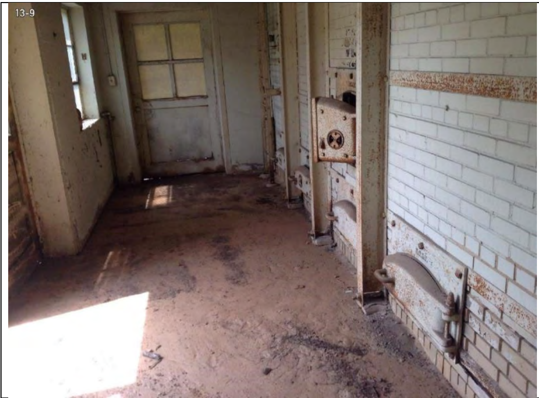
Photo 11-4 Ground level within incinerator building, cleanouts and dampers.
