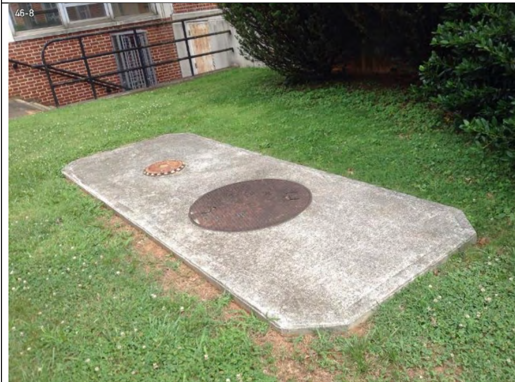
Photo 29-2 Close-up of 1,000-gallon diesel UST access, Building 46
