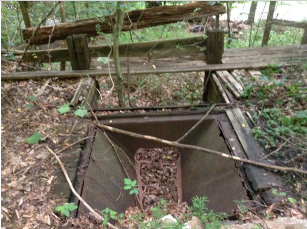
Photo 9-5 Remains of coal hopper at former rail siding used to deliver coal to facility, located east of Building 43 (old sewer treatment plant). No visual evidence of any remaining coal.
