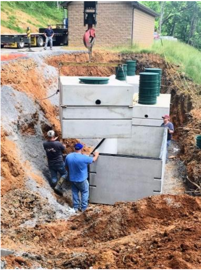
Left: Installation of settling tanks (2017).
