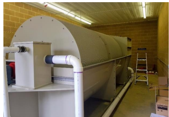
Top: Jeremy Weisman, CEO of EPC Middle: Cavitt's Creek, Tazewell; Bottom: EPC Waste Treatment Unit in Tazewell, Virginia
