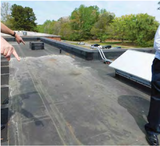
R3: LOW SLOPE MEMBRANE SYSTEMS, VIEW TO NORTH, EVIDENCE OF PONDING, (ABV RM 103 CEILING LEAKS) Photo 776
