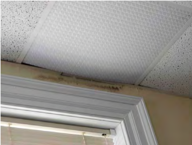
R5: CEILING FINISHES, CEILING TILE REPLACEMENT & WATER STAIN, DUE TO WATER INFILTRATION ABOVE WINDOW, RM 103A, Photo 744
