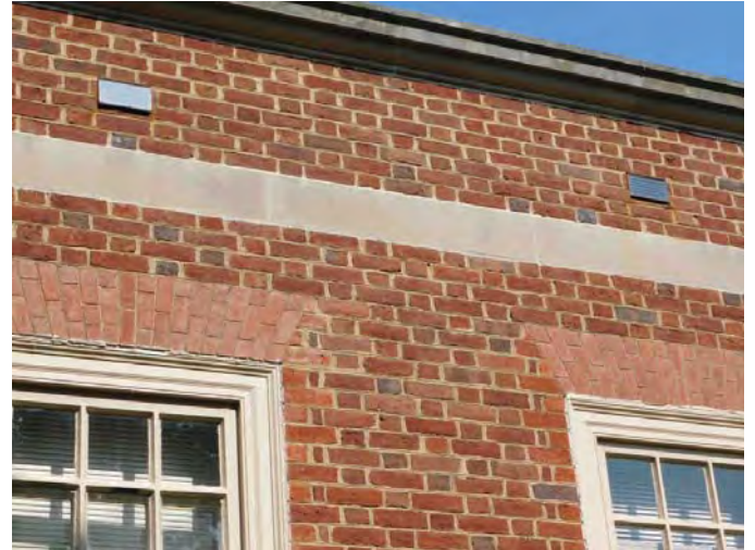
R1: BRICK VENT COVERS, ALL AROUND STRUCTURE, Photo 910
