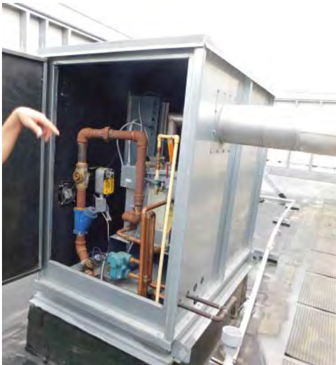
R3: REMOVE HUMIDIFIER NO LONGER IN USE. INSTALL HOSE BIB USING EXISTING PIPING, Photo 1560
