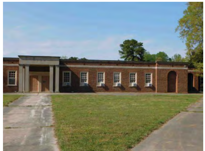
R15: WINDOW AC UNITS ON EAST SIDE, NEED CENTRAL AIR Photo 928
