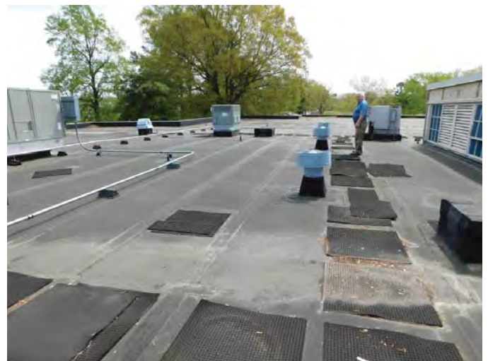
R3: LOW SLOPE MEMBRANE SYSTEMS, VIEW TO NORTH, EVIDENCE OF PONDING, Photo 785
