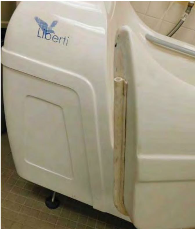
R1: LIBERTI TUB. TUBS LEAK THROUGH THE DOOR CLOSURE SEAL. Photo 2414
