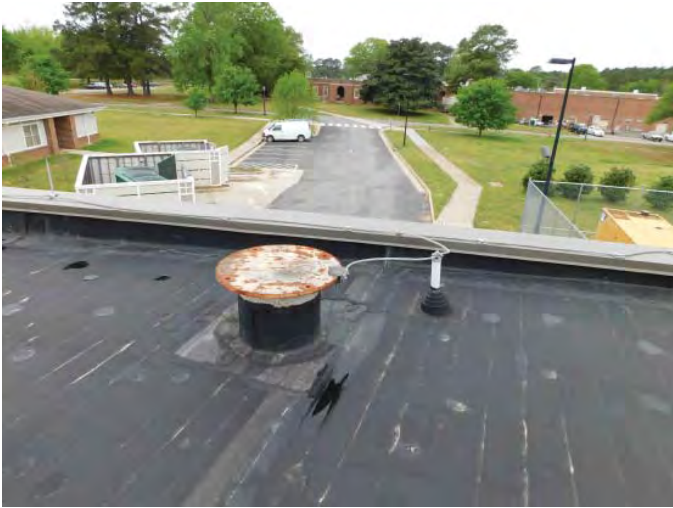
R6: JIB CRANE BASE ABOVE LOADING DOCK, Photo 1556
