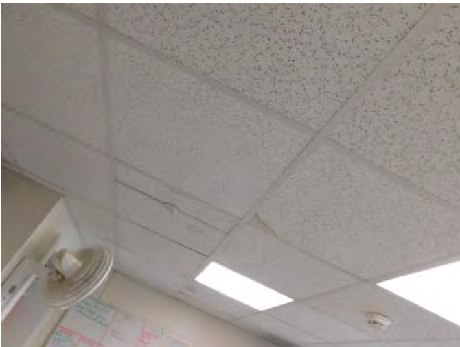
R8: ACOUSTICAL CEILING TILES, RM 317 Photo 202
