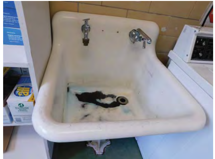
R11: LAUNDRY SINK RENEWAL, RM 247 Photo 2284
