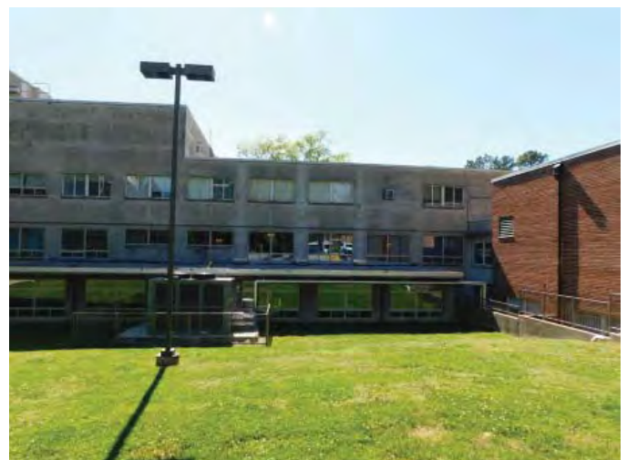
R4: WINDOWS, NORTH WING EAST EL Photo 759
