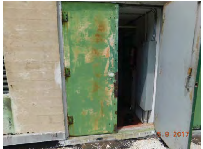
R6: EXTERIOR DOORS AND HARDWARE, PENTHOUSE, Photo 102c
