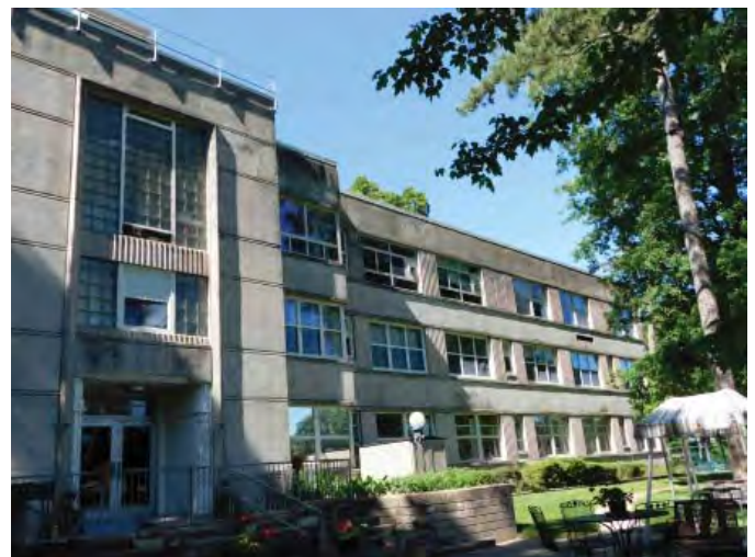
R4: WINDOWS, EAST WING SOUTH ELEV Photo 735
