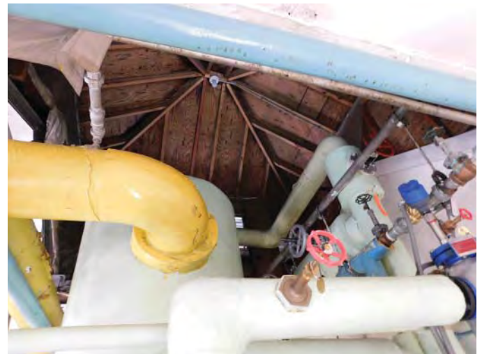
R13A: REMOVE & REPLACE ROOF ABOVE DA TANK, Photo SW 6013
