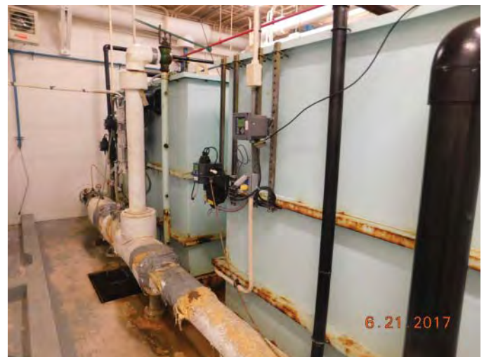
R20: REPLACE WATER TREATMENT PLANT FILTRATION TANKS, Photo 270
