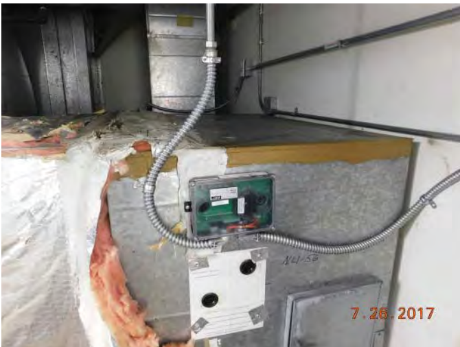
R6:DUCTS TO BE CLEANED, Photo SW 273
