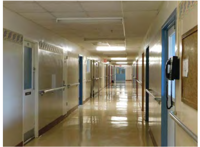
R8: RUBBER FLOOR REPLACE WITH EPOXY FLR, Photo 3442
