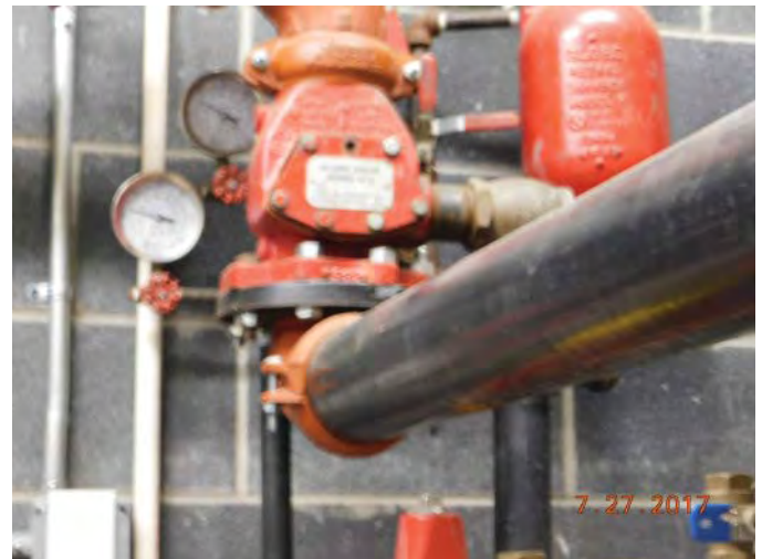
R7:PNEUMATIC CONTROLS, Photo SW 550
