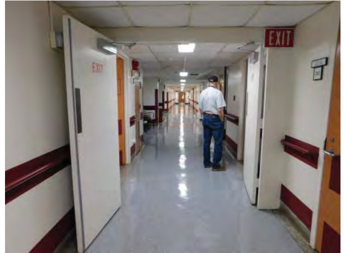
R7: ACOUSTICAL CEILING TILES, EAST WING CORRIDORS, Photo 48, FL 2
