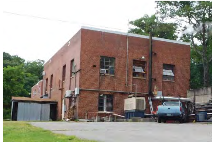
R18: REPLACE POWER PLANT DIESEL GENERATOR, Photo 255a
