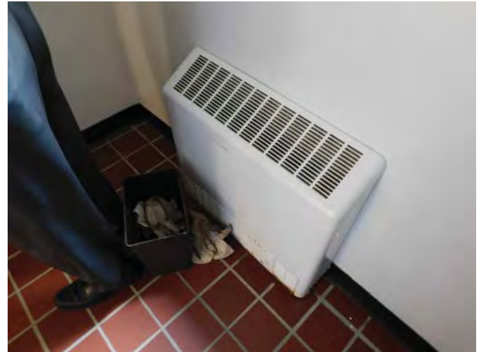
R16: FAN COIL UNIT REPLACE, RM 229 JANITOR'S CLOSET, Photo 2246,
