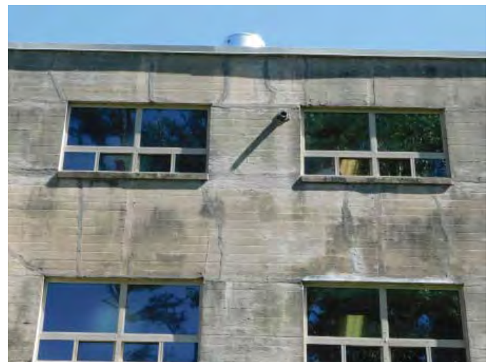
R2A: PRESSURE WASH EXTERIOR, Photo 653
