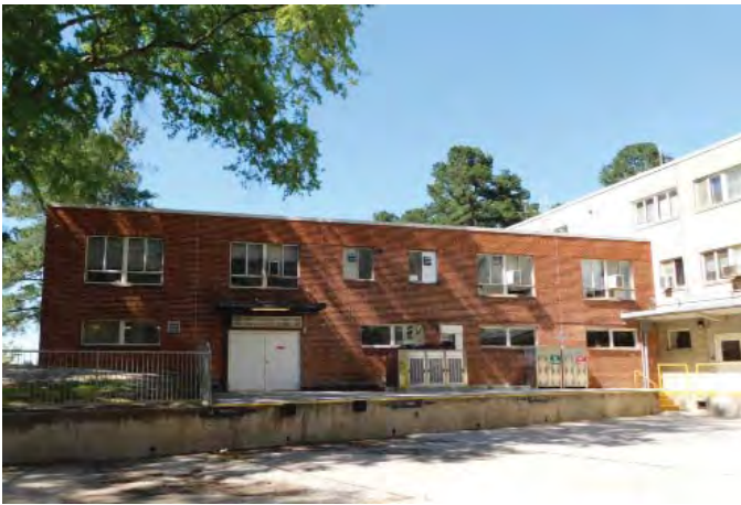
R4: WINDOWS, ADMIN SOUTH EL, & NORTH WING WEST ELEV, Photo 637
