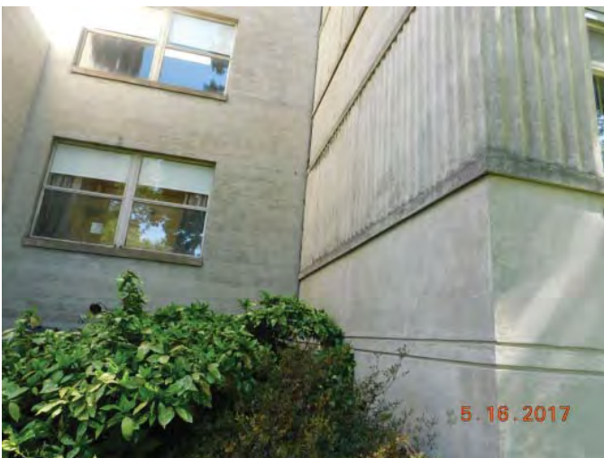
R3: CAULKING, EAST WING MEETS NORTH, ON SOUTH SIDE, Photo 545
