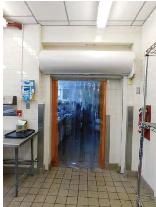
R4: ROLL-UP DOORS REPLACE W/ DOUBLE DOORS, Photo 1259
