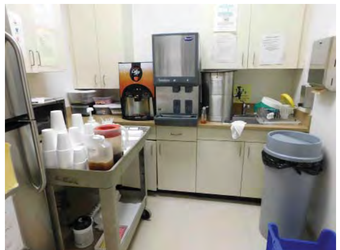
R5 NUTRITION ROOM NEEDING ADDITION COOL AIR, Photo 2011
