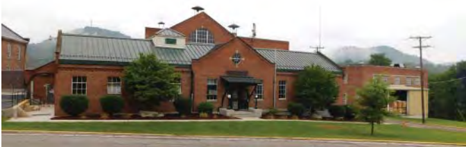
R13A: DA TANK, REMOVE & REPLACE ROOF ABOVE TANK ONLY
