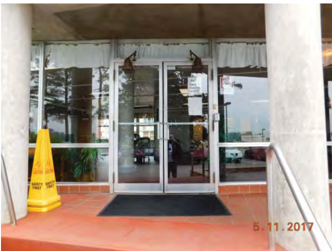
R6A: EXTERIOR DOORS STOREFRONT, MAIN ENTRY, Photo 219c
