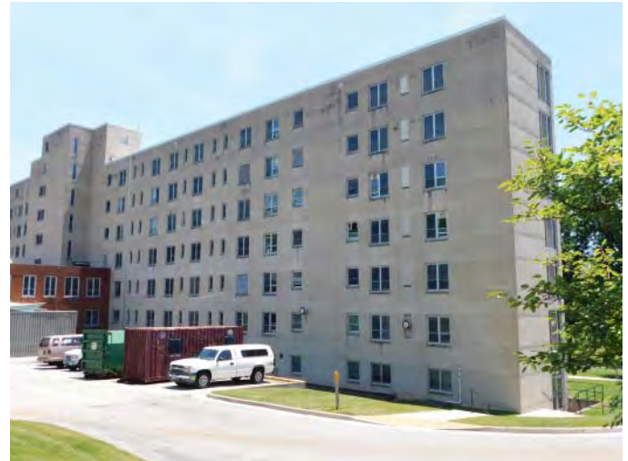
R2: EXTERIOR WALLS PRESSURE WASH REAR ELEVATION, Photo 4072
