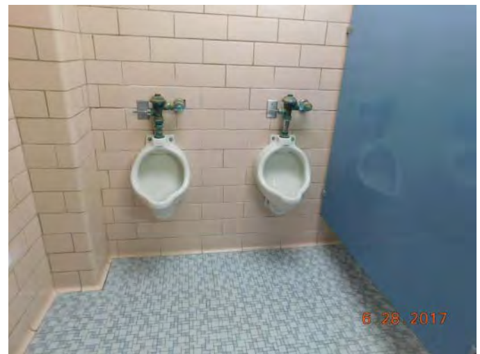
R9: WATER CLOSET RENEWAL- ROOM 109, Photo 819
