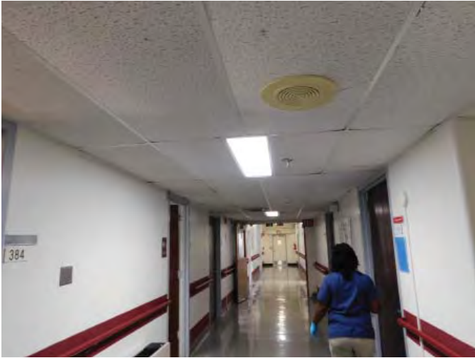
R7: ACOUSTICAL CEILING TILES, EAST WING CORRIDORS, Photo 49, FL 3
