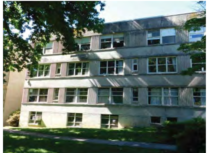
R4: WINDOWS, EAST WING SOUTH ELEV, Photo 706
