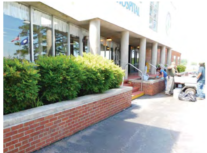
R6A: EXTERIOR DOORS STOREFRONT, MAIN ENTRY, Photo 003
