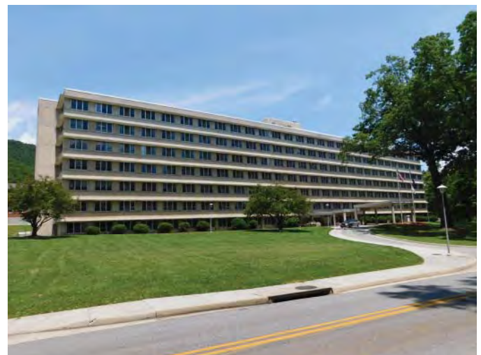
R2: EXTERIOR WALLS PRESSURE WASH FRONT ELEVATION, Photo 4091
