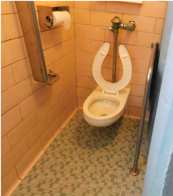
R10: WATER CLOSET RENEWAL- PATIENT FLOORS, Photo 327
