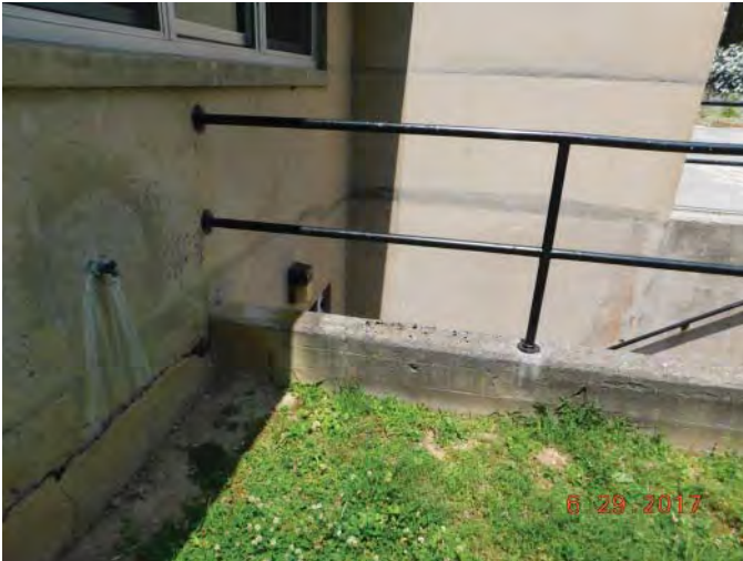
R1: STAIR RAILS, METAL, Photo 929
