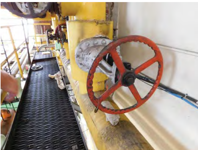
R10: DOMESTIC WATER DISTRIBUTION- VALVE HEADS 8" FLANGES REPLACE, Photo SW 5979
