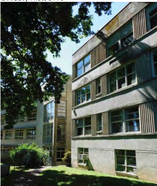
R2A: PRESSURE WASH EXTERIOR, Photo 711
