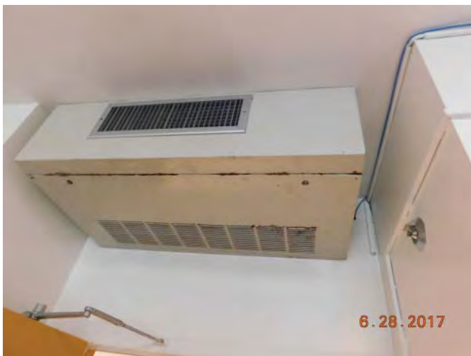
R16: FAN COIL UNIT REPLACE, RM 320, Photo 800
