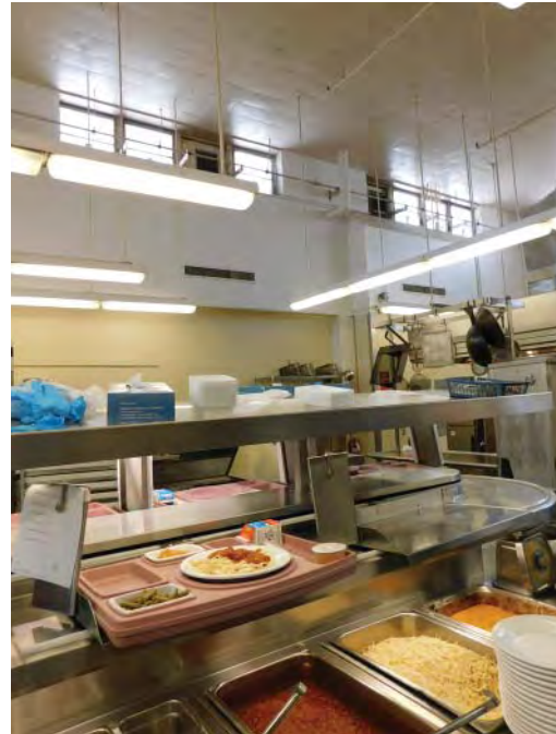
R14: EXHAUST SYSTEM FAN REPLACE, Photo SW 6944
