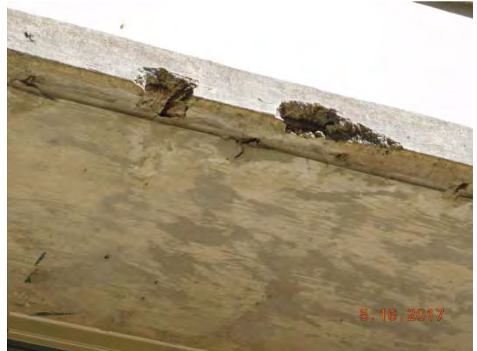
R2C: CONCRETE SHADE, WEST WING, SOUTH SIDE, Photo 535
