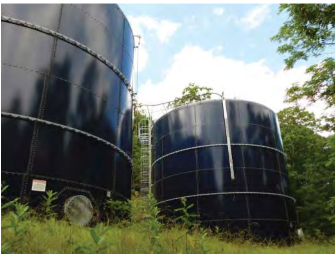
R21: RENOVATE ELEVATED WATER STORAGE TANKS, Photo 2118
