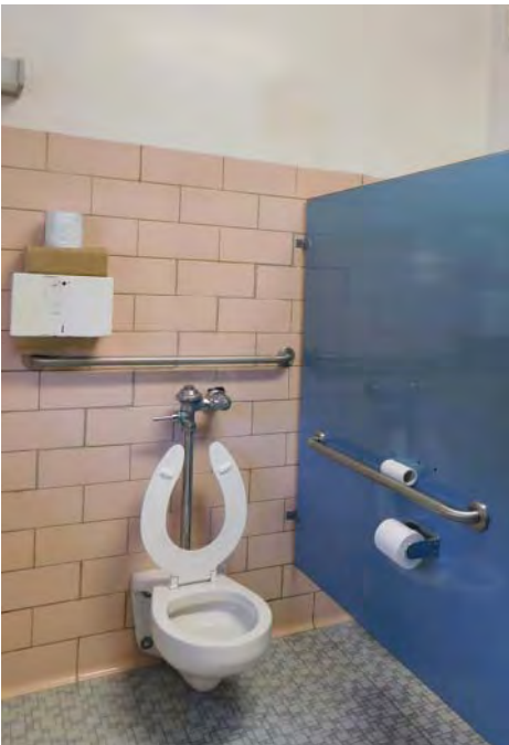
R9: WATER CLOSET RENEWAL- FIRST FLOOR, Photo 3974
