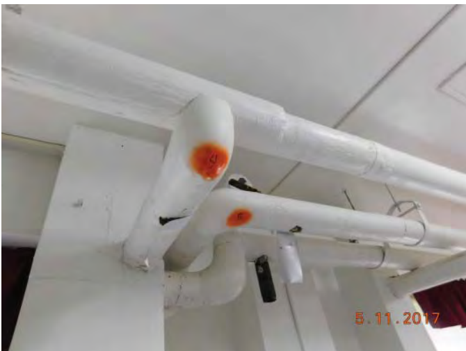
R11: EAST WING DRAIN, WASTE & VENT, EAST WING ONLY, FL 3, Photo 171
