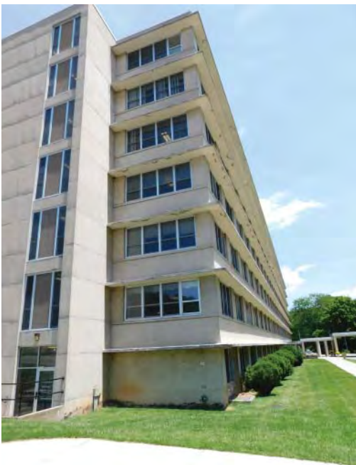
R2: EXTERIOR WALLS PRESSURE WASH WEST ELEVATION, Photo 4082
