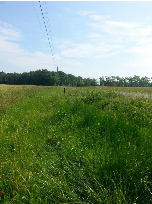
Bellevue Road 2-stage roadside ditch post-restoration June 2016.
