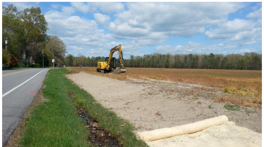
Glebe 2-stage roadside ditch during restoration, April 2015.
