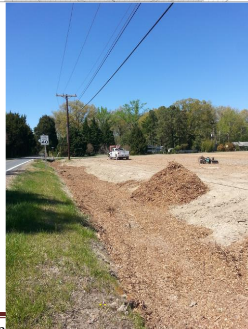
Unionville Wetland/Swale during restoration adding woodchips to enhance nutrient retention April 2016.
