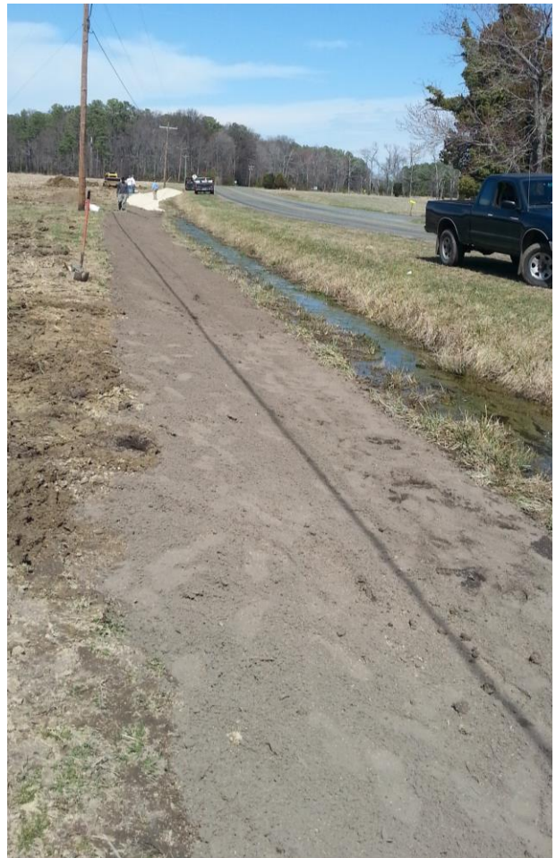
Adding top soil to wetland bench and side slope during construction.
