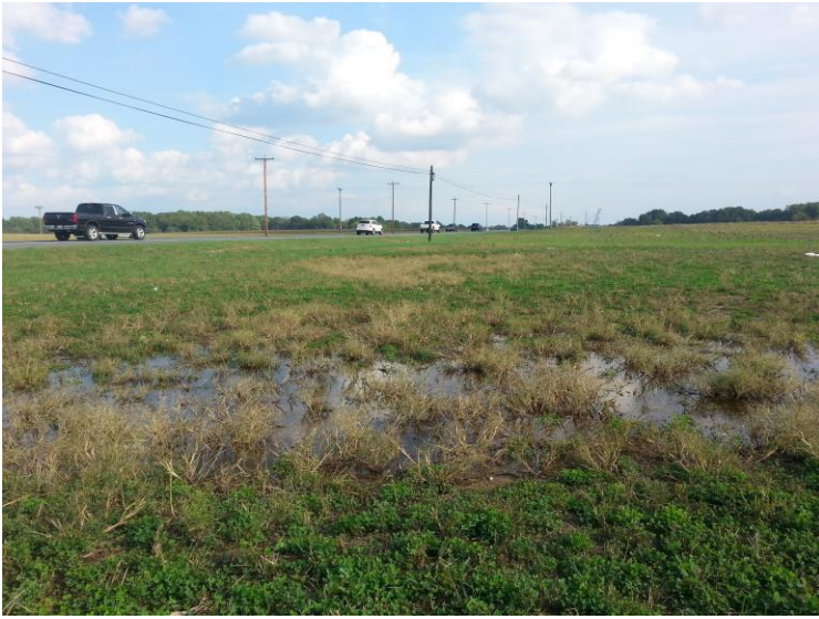
Dover Road wetland cell post-construction after a storm event.
