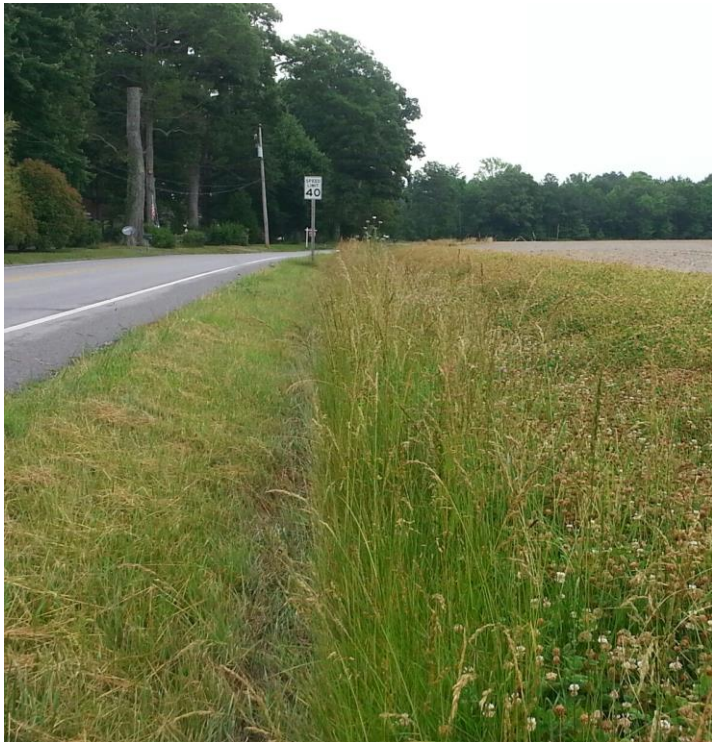
Glebe Road 2-stage ditch post-restoration June 2016.
