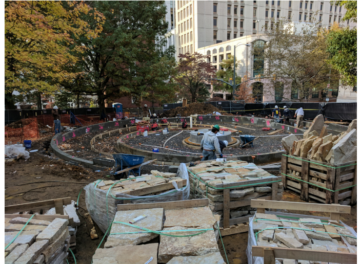
Construction of Mantle: Virginia Indian Tribute, fall 2017. Source: CSPC.
