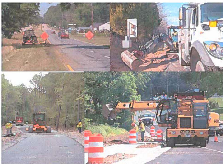
Figure 20 Routine Maintenance Operations
