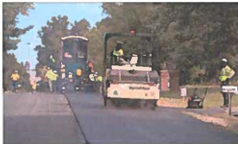
Thin Asphalt Mix
