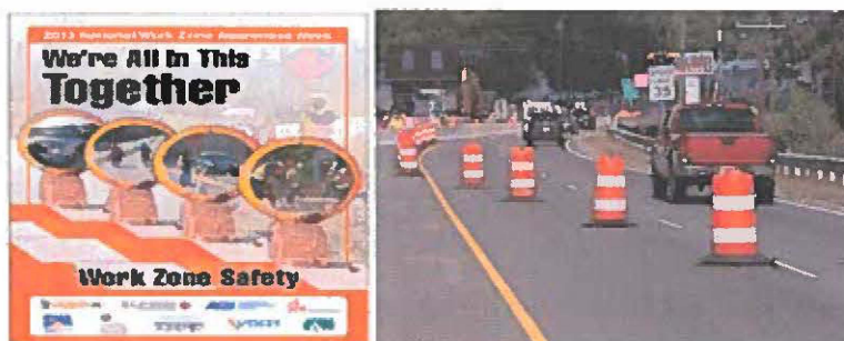
Figure 19: Traffic Safety Devices
