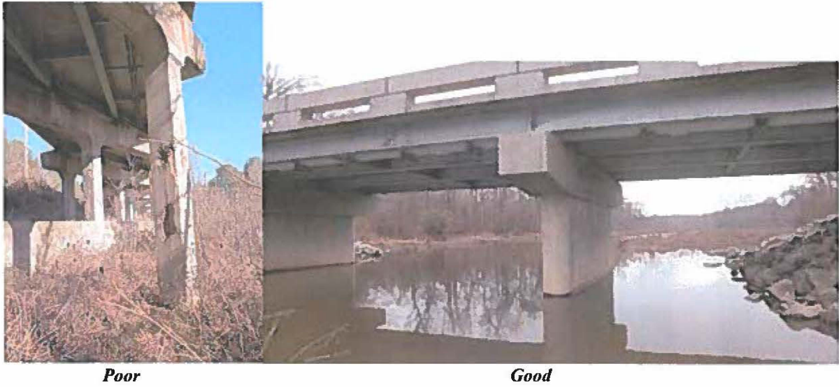
Figure 11: Comparison of Bridges in Poor and Good Conditions
