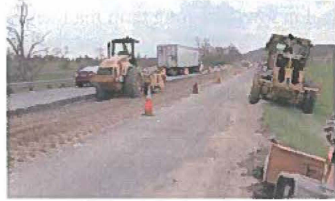
Full Depth Reclamation
