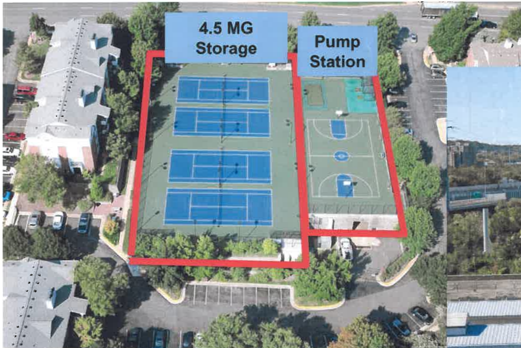
Tysons Corner: 4.5 MG Underground Tanks
