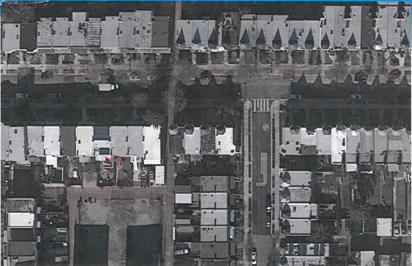
DC Water: After Shaft Construction
