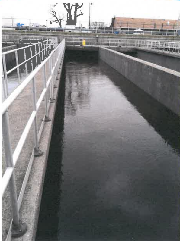
Easterly Plant, Cleveland, OH Chlorine Contact Tank
