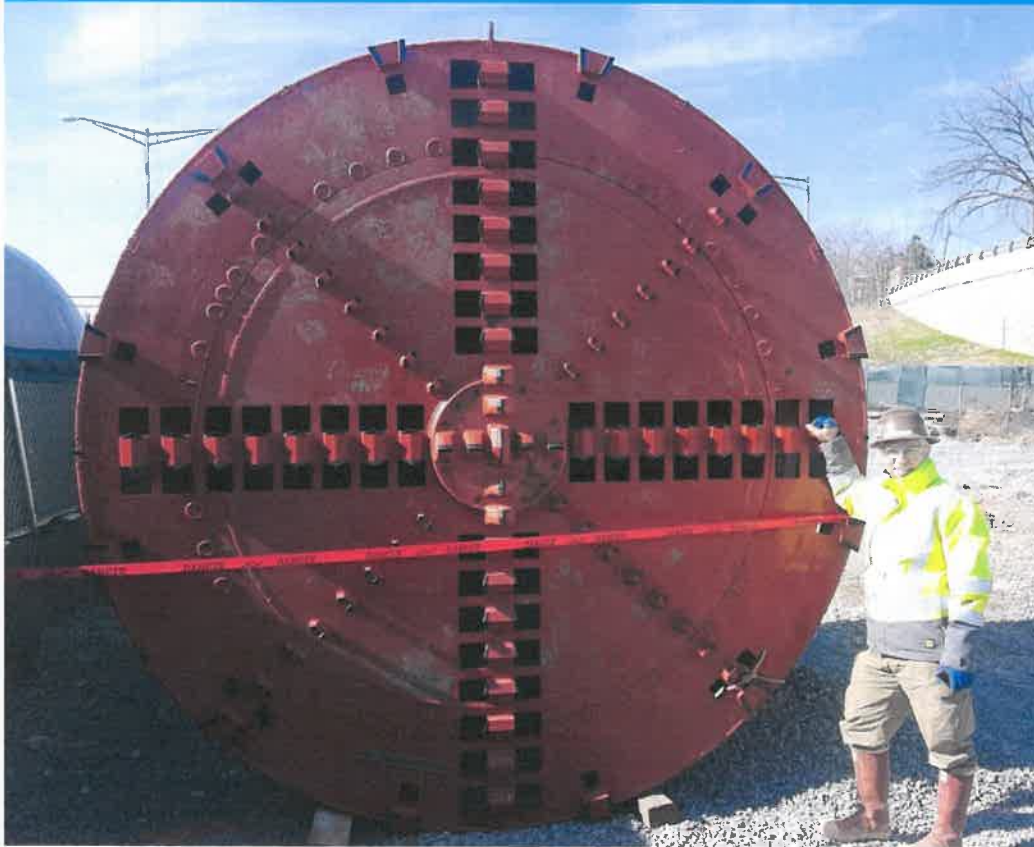
DC Water: 10-ft Diameter Tunnel Boring Machine and Finished Tunnel
