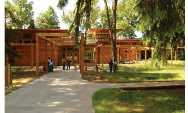
Figure 7.4 Bernheim Arboretum Visitors Center, KY Landscape/ building overlap; terrace and trellis structure provides focused building entry.
