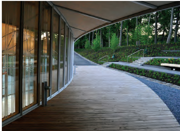
Figure 7.3 Brooklyn Botanic Garden Visitor Center, NY Shaded glazing and covered exterior space.
