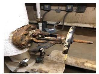
Corroded chilled water valve
