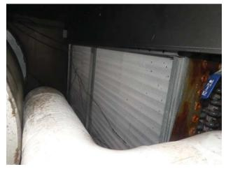
Inside one of the old roof top air handling units. The end of the chilled water coil is showing signs of rust and deterioration
