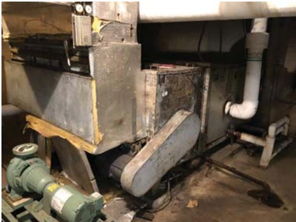
Air handling unit with damaged ductwork and insulation
