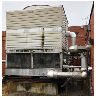
Cooling tower is in failing condition, as evidenced by leaks and algae growth
