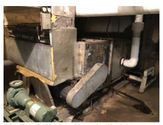
Air handling unit with damaged ductwork and insulation
