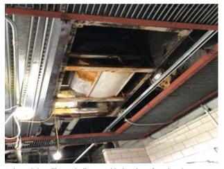
Indoor air handling unit disassembled and nonfunctional
