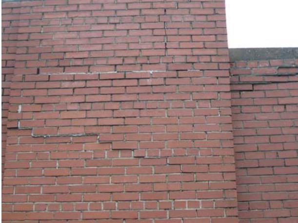
These photos depict the building's failing exterior wall conditions. The photos on the left show damaged masonry. The photos on the right show severe moisture damage.
