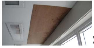
Ceiling collapse, temporary repair, staining on temporary repair near windows
