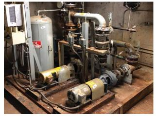
Hot water pumps and piping show visible signs of rust and deterioration
