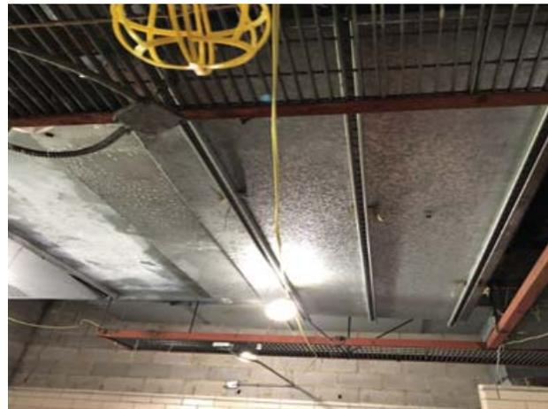
Indoor air handling unit with condensation forming on unit casing
