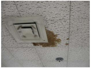
Interior ceiling damage due to duct insulation failure
