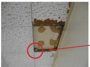
Interior ceiling damage due to duct masonry failure
