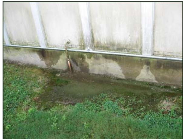
Apparent interior wall plumbing issue resulting in damage and mold on foundation wall
