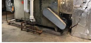
Dry rotted flexible duct connector
