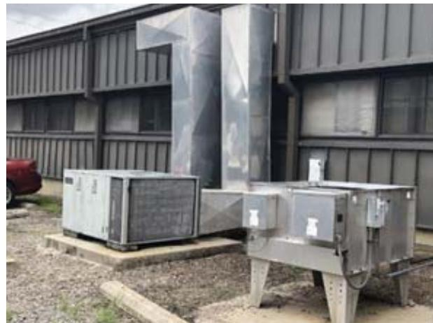
Grade mounted air handler and computer room air conditioner condensing unit
