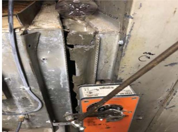
Dry rotted flexible duct connector
