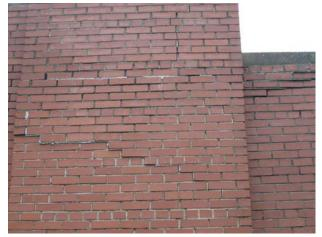
These photos depict the building's failing exterior wall conditions. The photos on the left show damaged masonry. The photos on the right show sever moisture damage.
