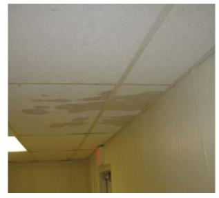
Typical condition throughout the building, water staining on ceiling tile
