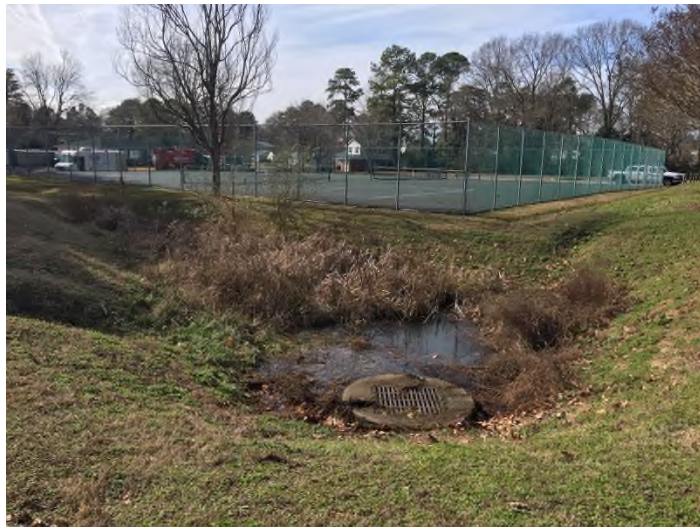
Figure 2.39. Image of stormwater retention basin upland from DO-1. Connectivity with the DO-1 outlet in Buchanan Creek is uncertain.
