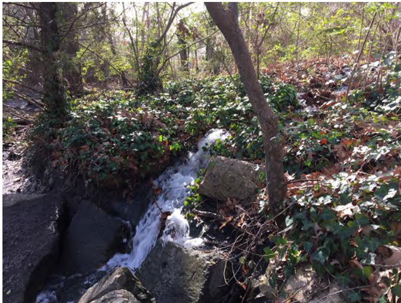
Figure 2.41. Image of unmarked discharge pipe during January 23, 2019 sampling survey.
