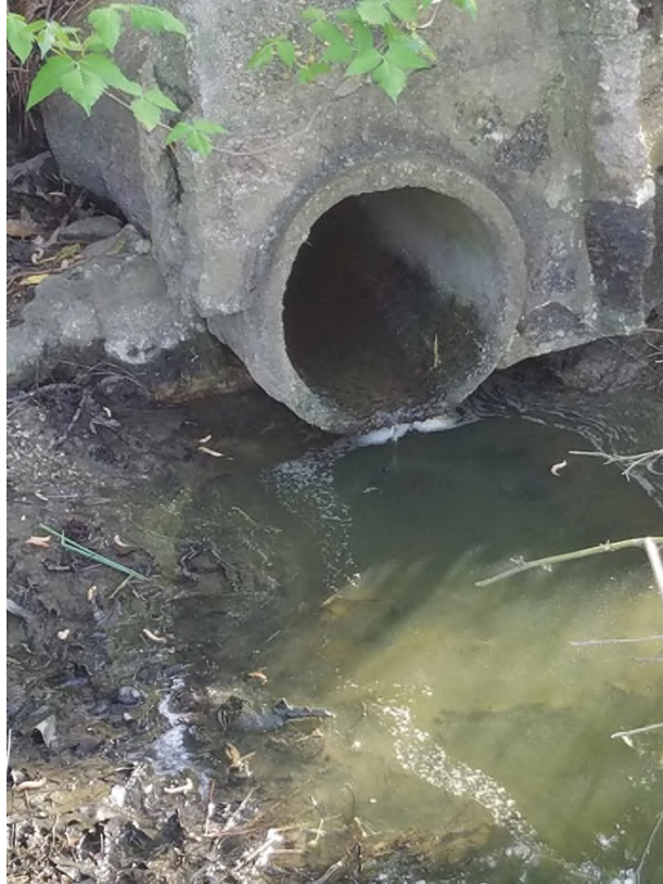
Figure 2.40. Image of DO-3. Flow rate is estimated at 200 ml/sec.
