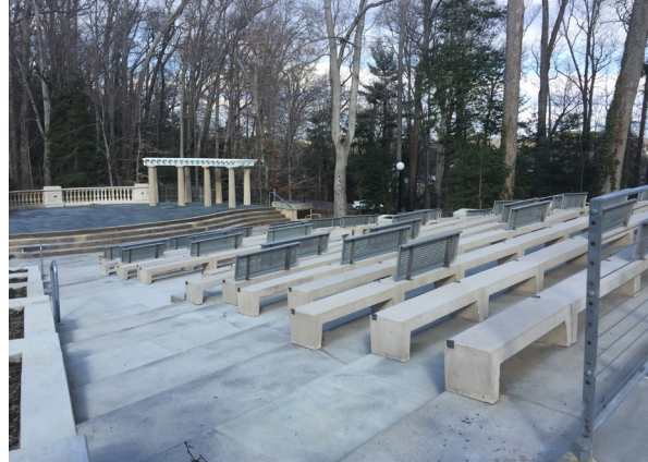
UMW's Amphitheater after restoration.
