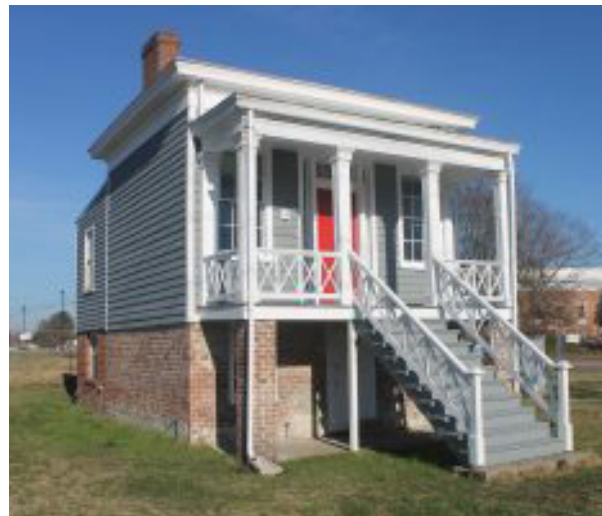
VSU's Summerseat after the first phase of restoration completed in October 2016. (Photo: HistoriCorps)
