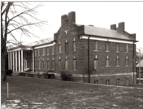
An administration building at Virginia Correctional Center for Women.
