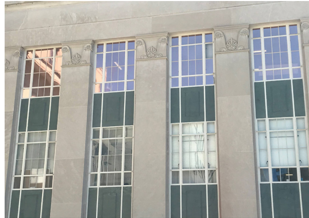
Top: VDOT's Central Highway Building and a close-up view (above) of its window restoration, which retained the historic character-defining elements of the original design.
