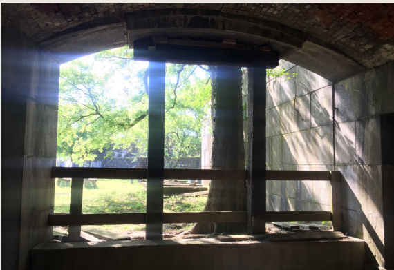
Timber bracing supporting the casement in silhouette.
