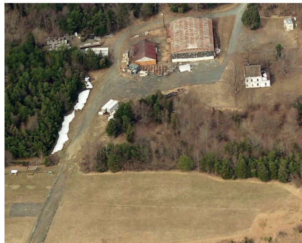
A circa 2010 aerial view looking west at Milton Field, a pre-WW II complex. (Photo: Paul Freeman)
