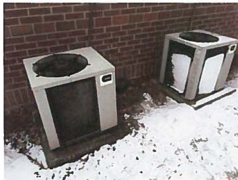
Ice build-up on the existing HVAC units indicated the units were not operating efficiently
