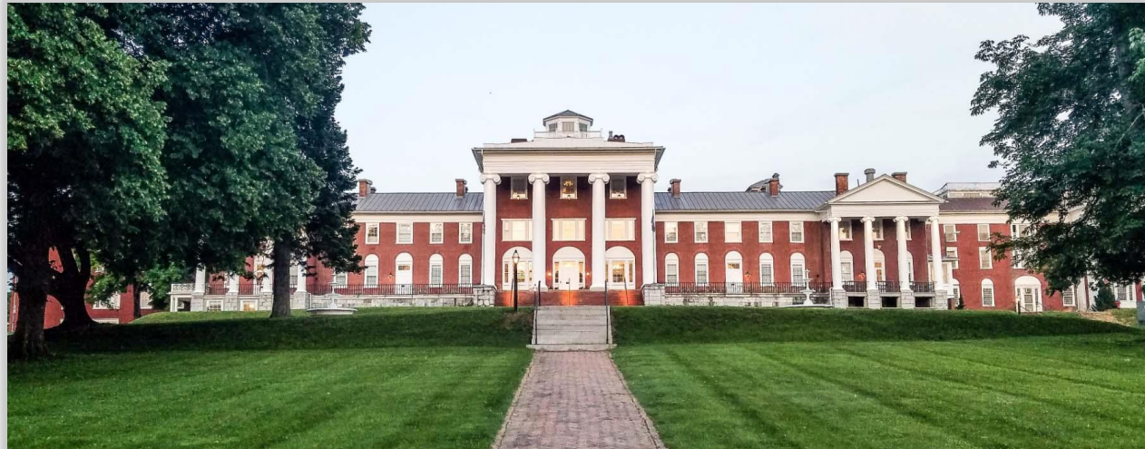
Blackburn Inn LLC, City of Staunton
