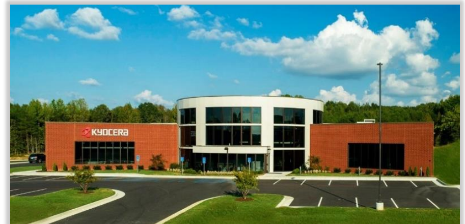
Kyocera SGS Tech Hub LLC, City of Danville
