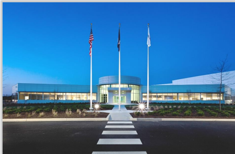
Rolls-Royce Crosspointe LLC, Prince George County
