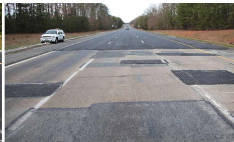
Poor/Fair Pavement Being Restored
