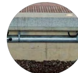
West Falls Church Platform After Improvements
