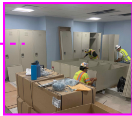
New Locker Room Assembly
