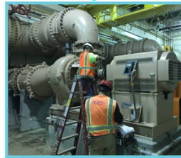
Primary Effluent Pump Replacement
