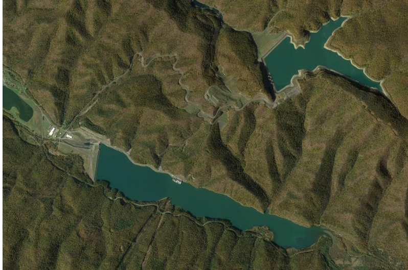
Figure 5. Bird's eye view of the Bath County pumped hydro facility.
