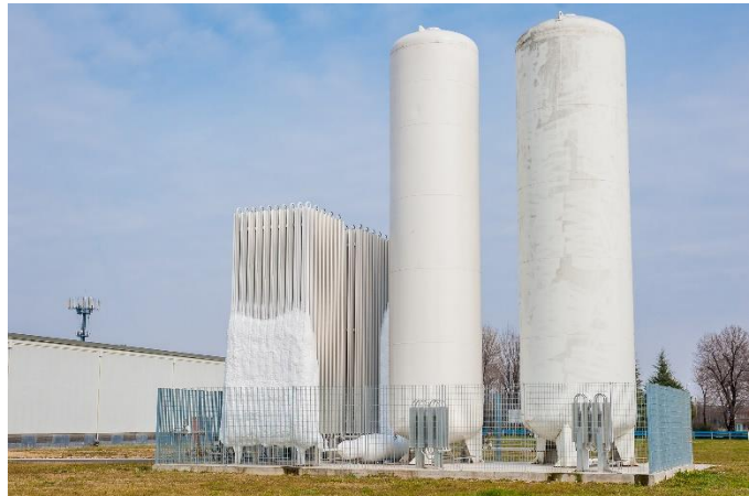
Figure 9. This image shows liquid oxygen stored in above ground silos. LAES systems can store their liquid-air storage medium in similar tanks.
