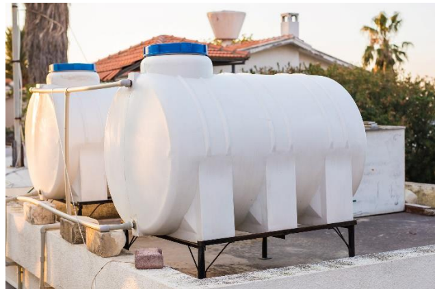
Figure 11. Tanks like these can be installed on commercial and residential properties to store water heated by electricity or the sun. This simple form of energy storage uses this water at a later time to reduce heating loads.
