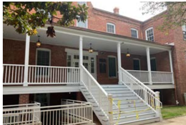
Vawter Hall porch during restoration.
