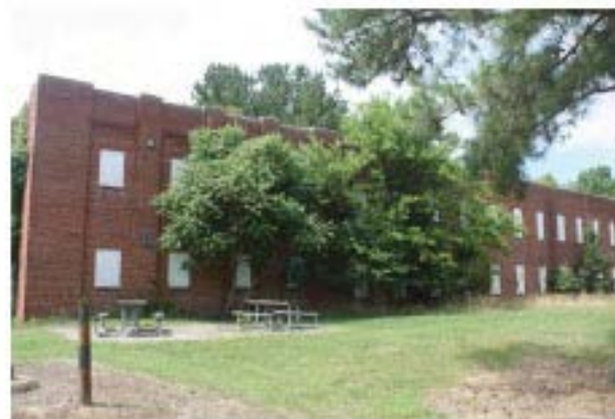
Eastview 1936 Wing Rear Façade, view looking northeast.
