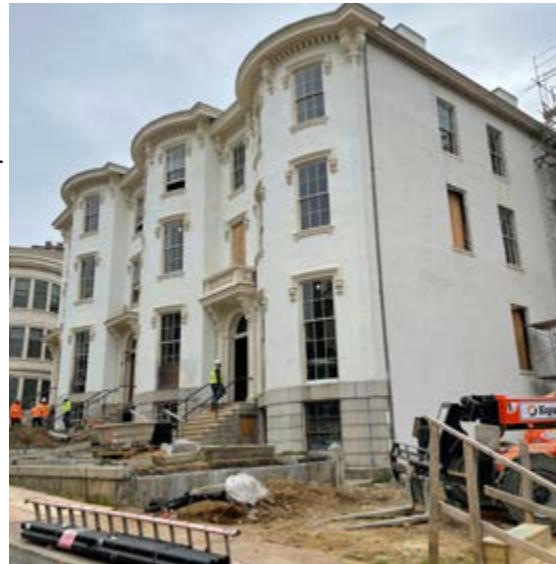
Morson's Row undergoing rehabilitation.
