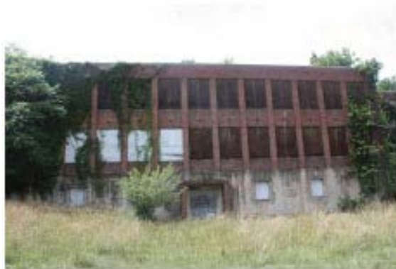
Eastview Rear Façade Center Portion Loading Dock, view looking north.
