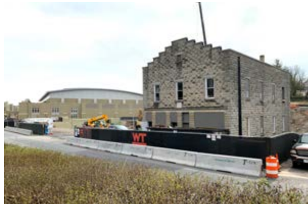
VMI proposes to re-purpose the American Legion building. (Photo: Kjellstrom + Lee)
