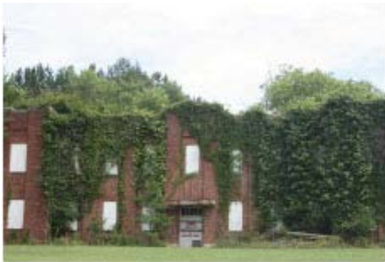
Eastview 1936 Wing North Façade, view looking south.
