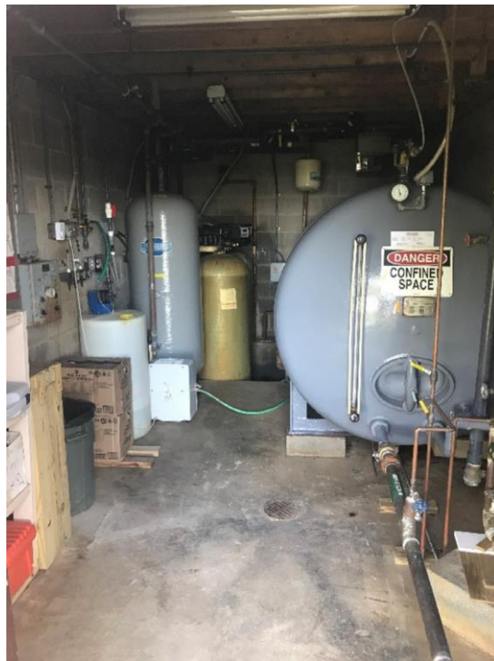
Photograph 2 – Interior of Well House
