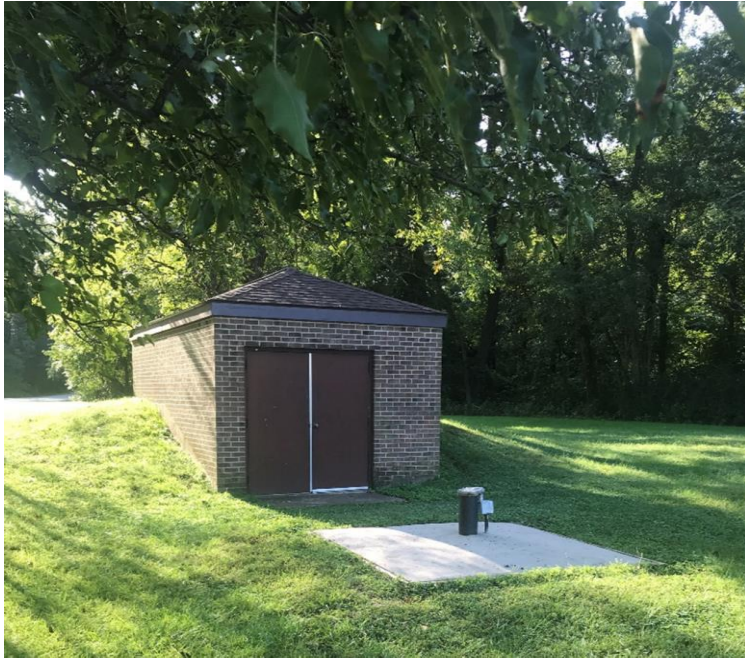
Photograph 1 – Well House & Well
