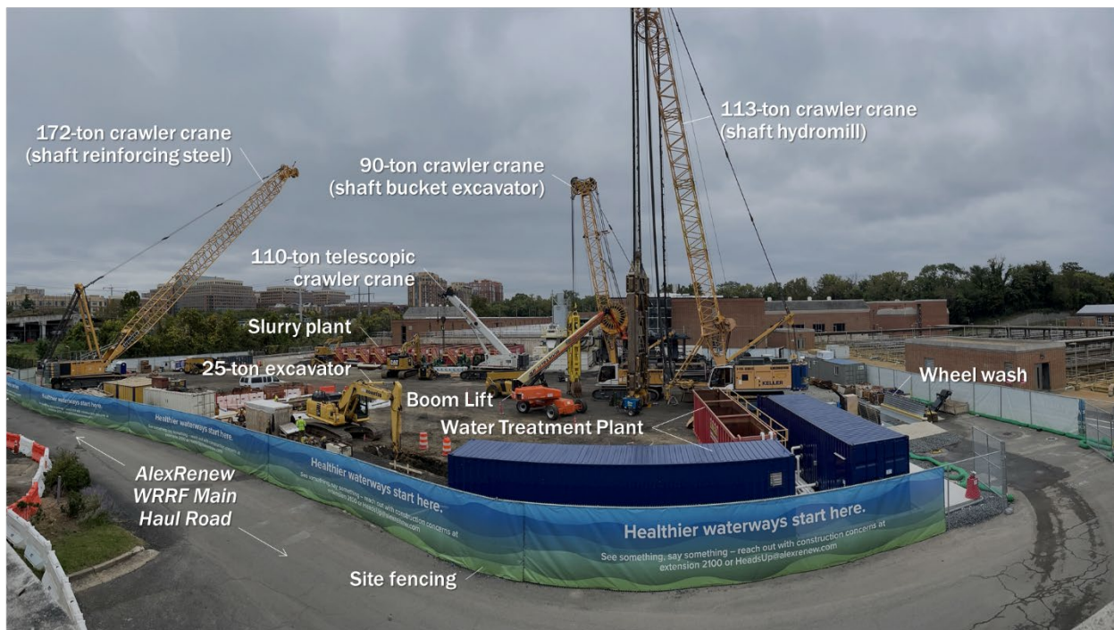
Figure 3. AlexRenew Construction Staging Area, readying for shaft construction on October 12, 2021
