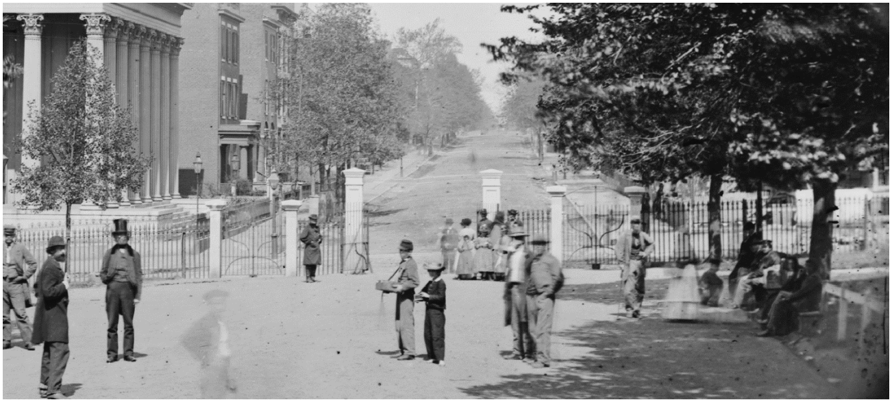
(detail showing the original Sabbaton Fence and Gate at 9 th and Grace Streets), John Reekie, "Richmond, Virginia. St. Paul's Episcopal Church. (Grace Street)," c. 1865, Library of Congress, LC-B815- 937 [P&P]
