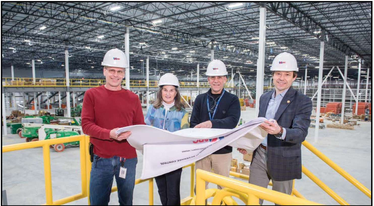
ABOVE: Chief Retail Operations Officer Mark Dunham, Board Chair Maria Everett, Project Manager Chris Porras and CEO Travis Hill tour the 315,000-square-foot distribution center. Hard hats and closed toes shoes were a requirement during the construction phase. Photo by Doug Buerlein Photography, courtesy of StateWays Magazine
