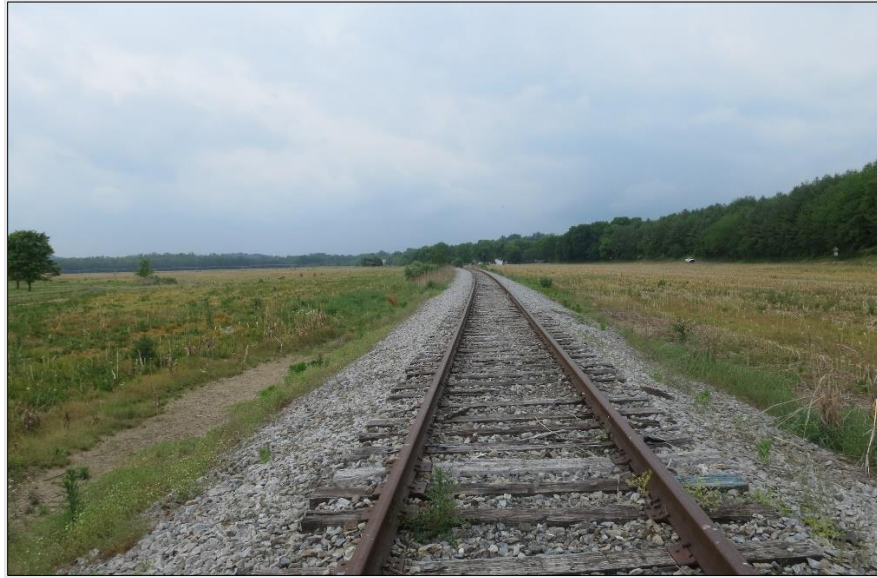
Figure 9: North of Town of Timberville
