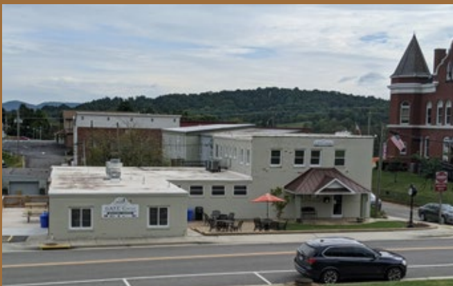
The Grayson Agricultural and Technical Education Center (GATE Center) in Grayson County has transformed the former County Sheriff's office into offices for Virginia Cooperative Extension, an agribusiness incubator, and a Financial Stability Center serving both the county and the region.
