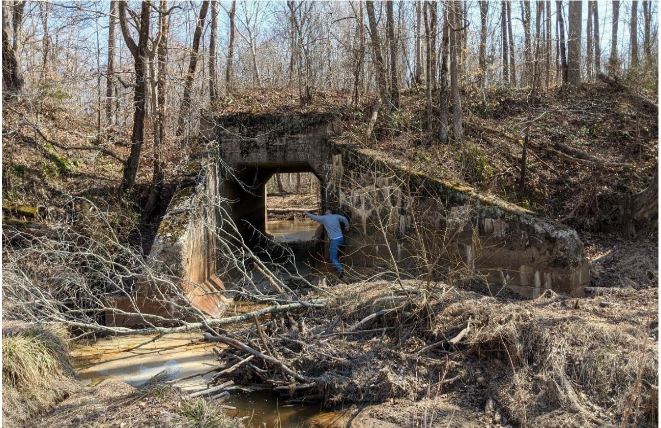
Figure 23 - A culvert that needs repair at milepost 6
