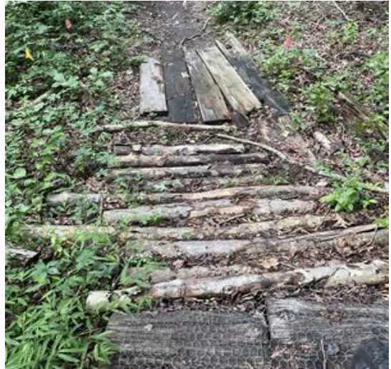
Figure 18 - Existing planks over wet areas along the Trail
