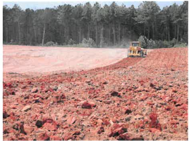
FIG 2 – Final deep ripping of reconstructed soil profile following topsoil return. This practice was originally added in 2004 to rid the subsoil of grading related compaction and to enhance crop rooting and water infiltration. The practice was modified in later years to be applied after topsoil return in certain instances, but is routinely applied to the subsoil materials following application of lime and P fertiliser (photo: C Zimmerman).
