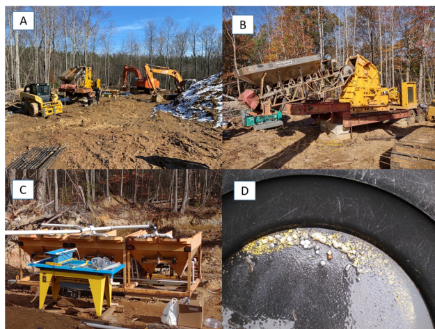
FIGURE 1-5 Photographs of Moss Mine reclamation site, Goochland County, Virginia. (A) Photograph of some of the equipment used to collect rock and sediment materials for reprocessing. (B) Photograph of the crusher being used to process waste material at the Moss Mine. (C) Three jigs used to capture mercury, gold, and lead. (D) Recovered gold and mercury from the Moss Mine site.
