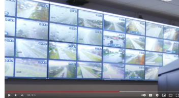
Traffic Operations Center/ Customer Service Center
