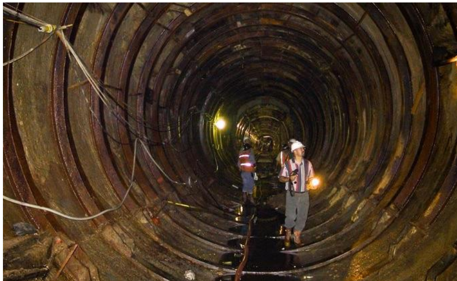
Figure 6. Richmond’s 14-ft Diameter Hampton-McCloy Tunnel
