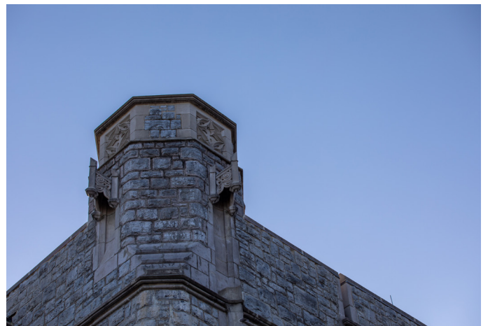
Pictured: (Above) Holden Hall's 1939 south wing faces the Drillfield, the center of campus. It is an excellent example of Carneal, Johnston & Wright's collegiate gothic compositions at Virginia Tech. (Bottom left) A restored precast window surround and replacement steel window. (Bottom right) A small octagonal turret with architectural precast details, providing vertical emphasis to the southeast corner of the building, punctuating the façade and announcing the entry point. Photos courtesy of Virginia Tech.
