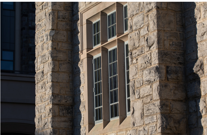
Pictured: (Above) Holden Hall's 1939 south wing faces the Drillfield, the center of campus. It is an excellent example of Carneal, Johnston & Wright's collegiate gothic compositions at Virginia Tech. (Bottom left) A restored precast window surround and replacement steel window. (Bottom right) A small octagonal turret with architectural precast details, providing vertical emphasis to the southeast corner of the building, punctuating the façade and announcing the entry point. Photos courtesy of Virginia Tech.
