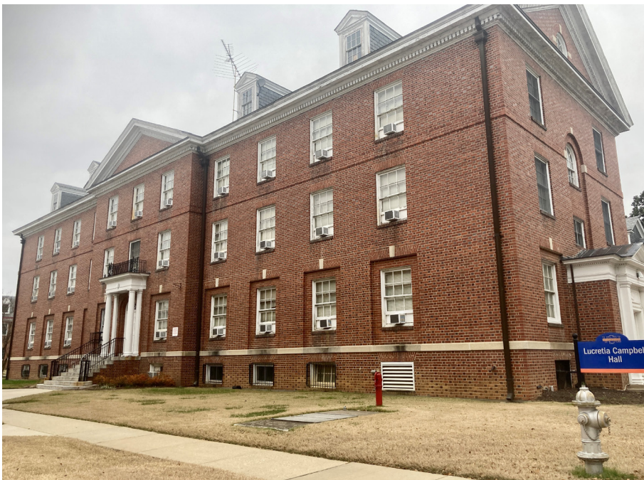
Pictured left: Lucretia Campbell Hall on the VSU campus in 2023.
