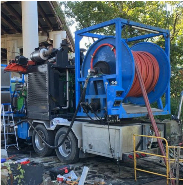
Shockoe 96-Inch Interceptor and Twin 66-Inch Siphon cleaning
