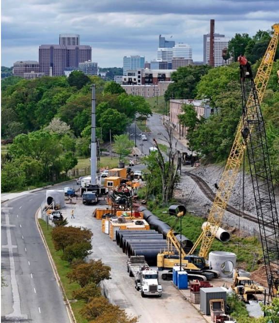
Construction of Outfall 004 Interim Plan Project
