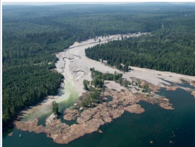
Mount Polley tailings dam failure. Image courtesy: Jonathan Hayward
