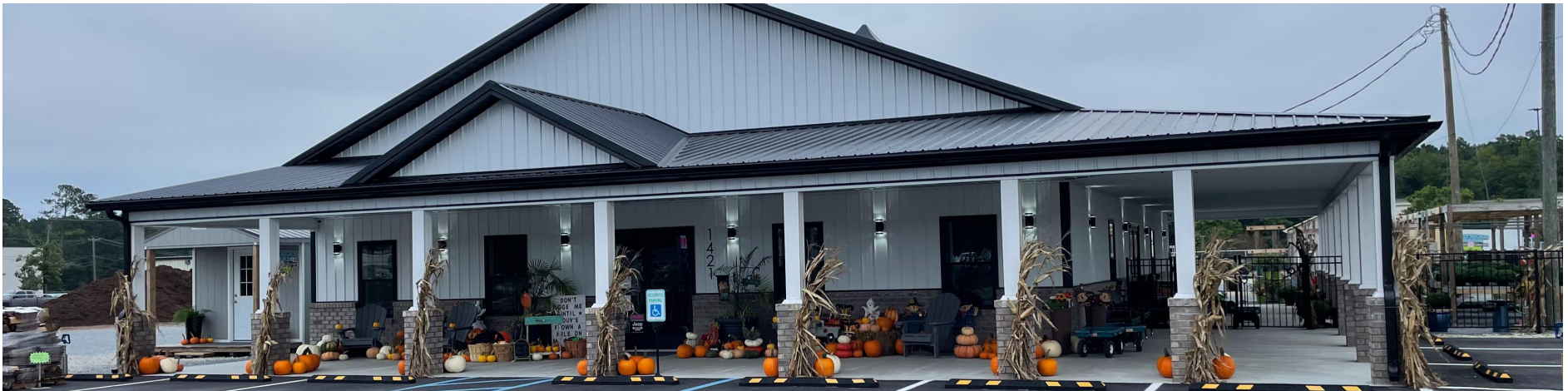
Southern Charm Garden Center, located in Franklin, VA is a retail nursery and garden center expansion that included a new 3,000 square-foot wood framed, metal single story building, as well as improvements to an existing metal warehouse structure.
