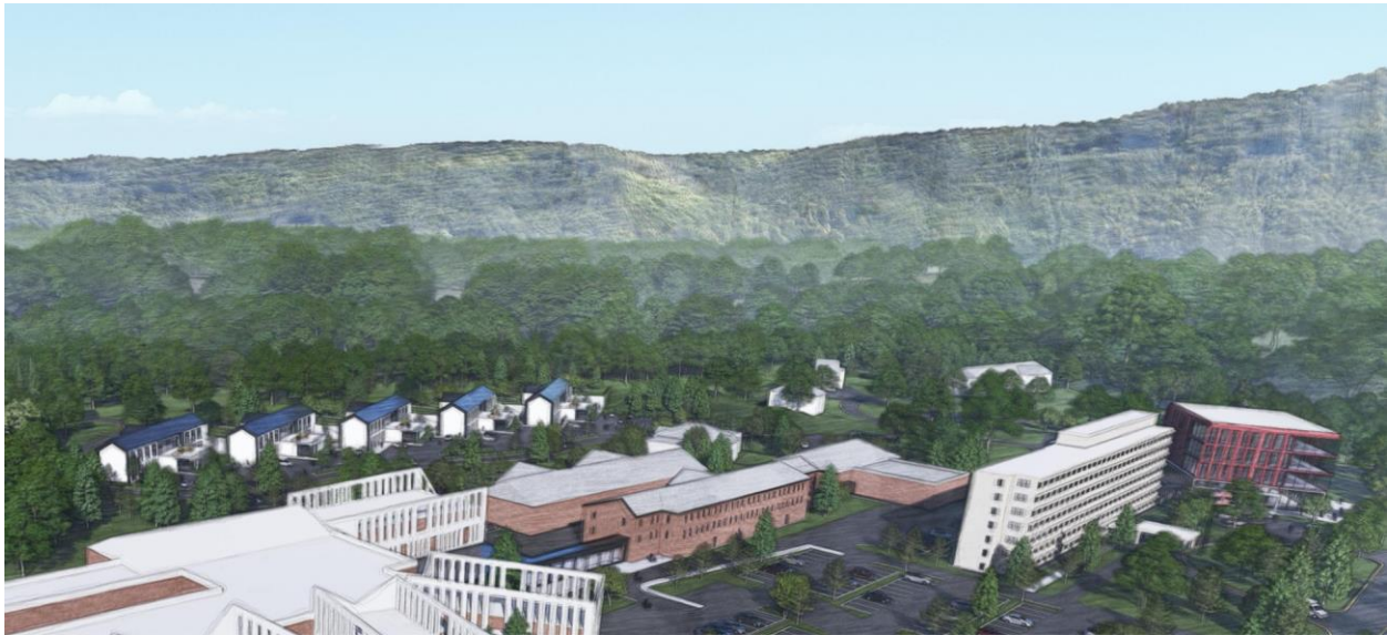
SUD Outpatient Building, SUD Inpatient, SUD Residential Housing surrounding Catawba Hospital looking Northeast - Option C
