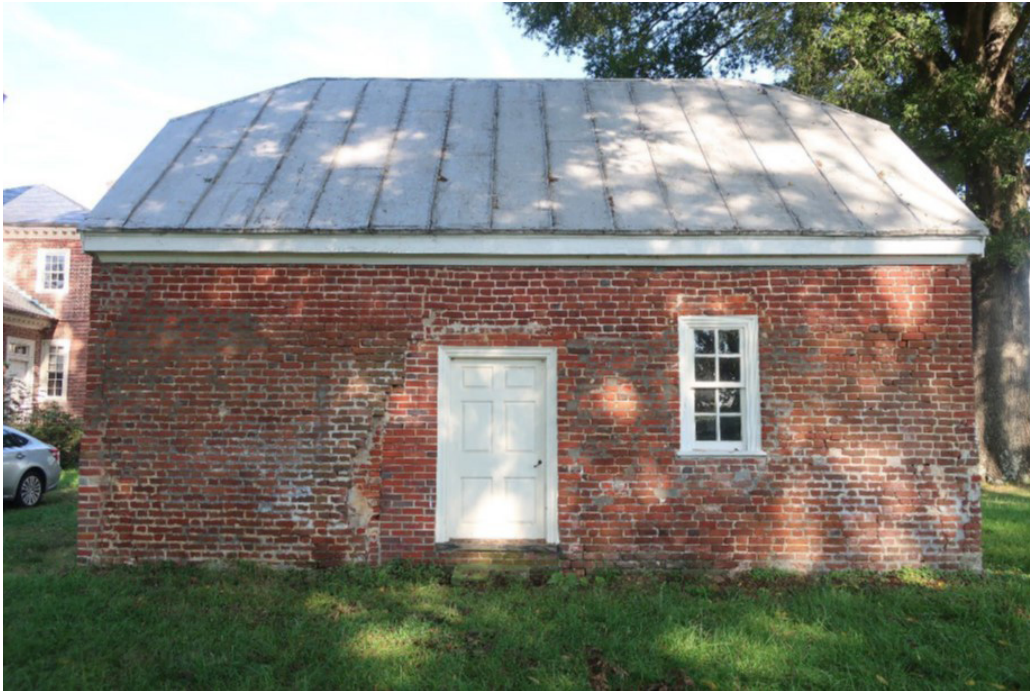
The Belle Isle circa-1760 summer kitchen: before work, the south elevation showing improper repointing and to the left, where brick is pulling away from the wall. Additionally, see the replacement brick at door.
