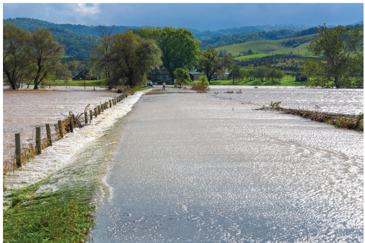
RURAL ROAD FLOODED IN GRAYSON COUNTY, VA FROM HURRICANE HELENE
