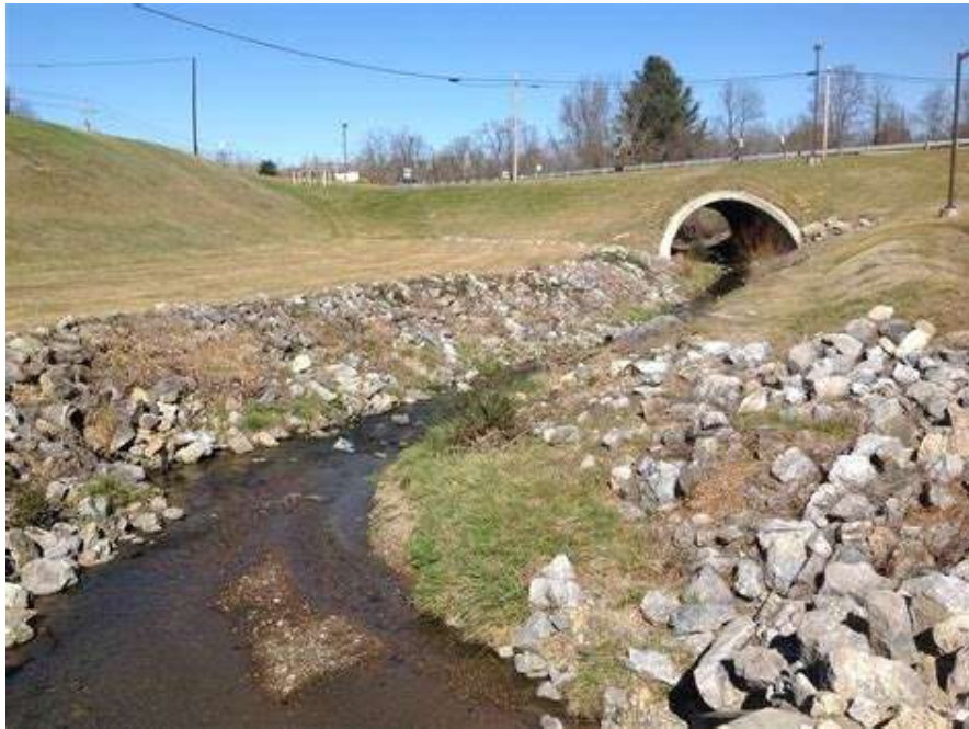
Figure 1 - Towne Branch stream restoration helps reduce erosion and protect local waterways.
