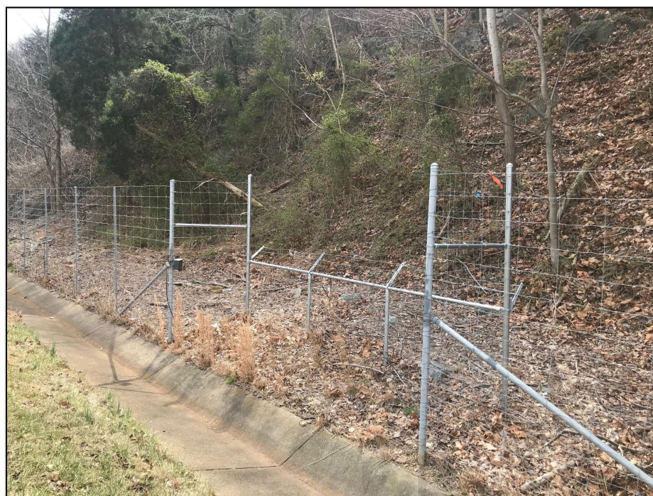
Figure 2-12. A wildlife jump-out located along I-64 in Virginia. (Donaldson and Elliott 2021)
