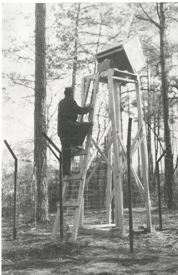
(a) Monitoring well near Franklin, Virginia, in 1941. Water levels rose to about 7 feet above land surface when the well was first installed to a depth of 600 feet below land surface.
